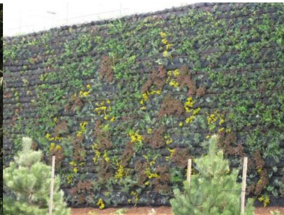
Green wall of soil filled geotextile fabric bags is tied back into the slope
