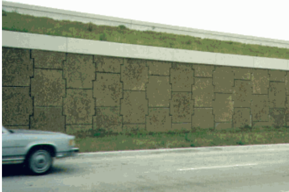
FIGURE 8-19 WALL FACE PANELS
