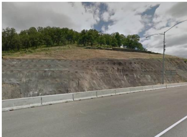
FIGURE 8-6 SHOTCRETE AND SOIL NAIL WALL ON I-5
