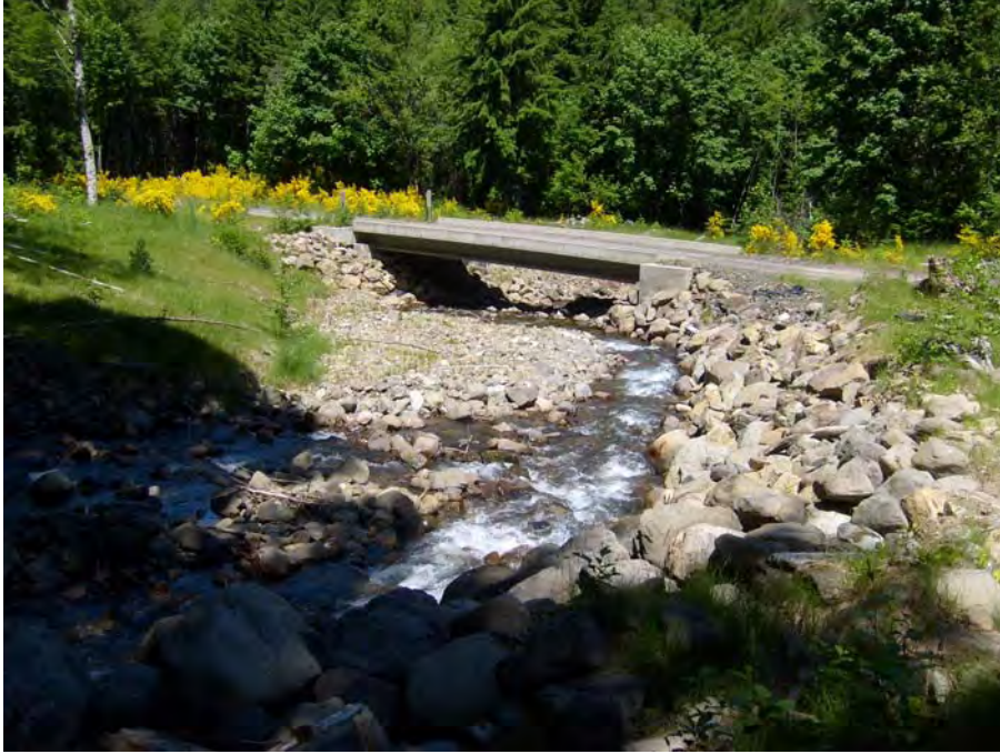
Figure 6-7. Aggradation upstream of a small creek in rural King County, Washington. Herrera Environmental Consultants.
