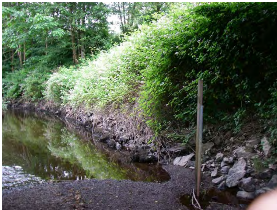
Figure 6-10. Blackberry covered riprapped bank near Mt. Vernon, Washington. Herrera Environmental Consultants.
