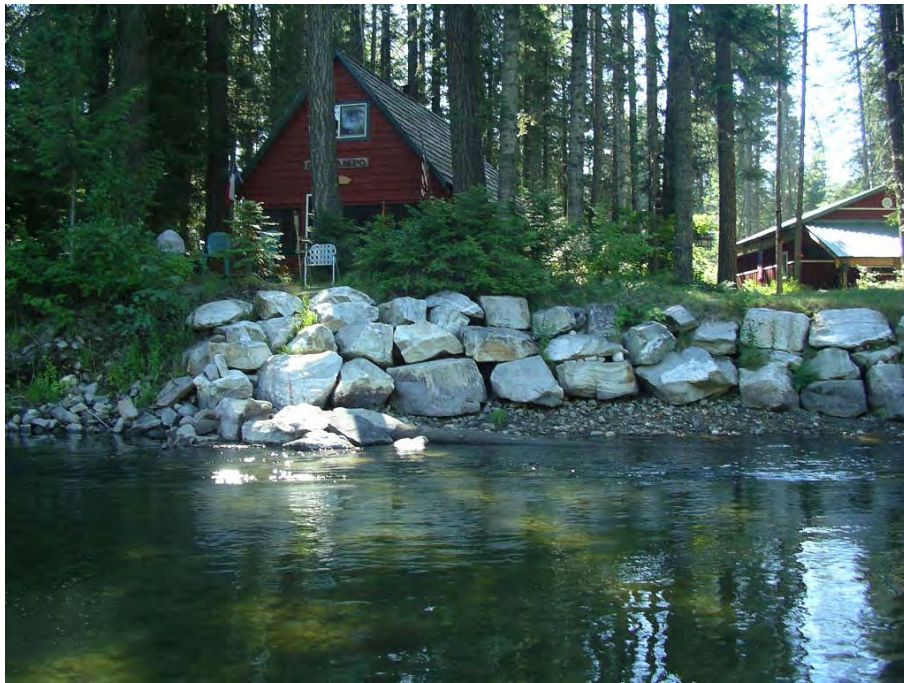
Figure 6-8. Riprap along the Wenatchee River in rural Chelan County, Washington. Herrera Environmental Consultants.
