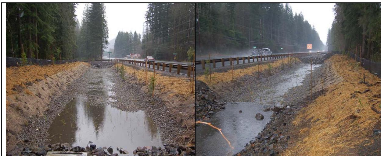
**Figure 1 Extended detention dry pond**
