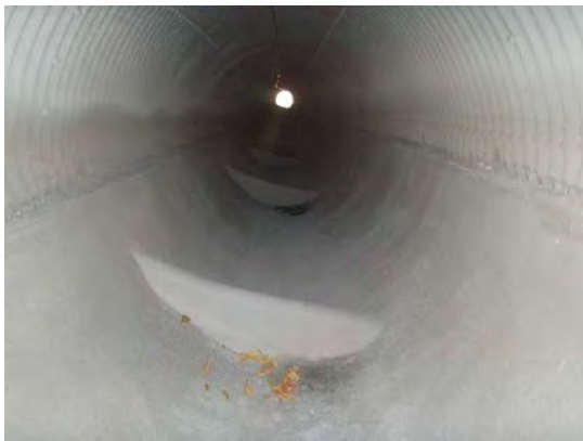
Invert paving with sloped weirs prior to the return of flow (9/20/16)
