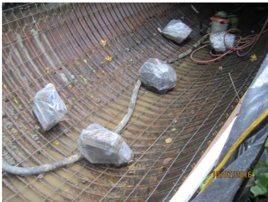
Rebar cage and fish rocks in place prior to invert paving (10/7/16)
