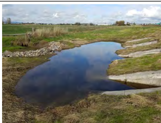
Culvert outlets with weir
