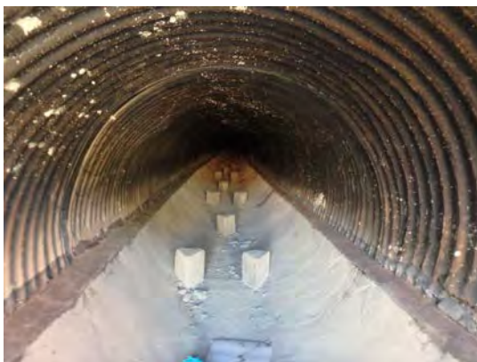
Inside culvert showing invert paving and roughness features (9/20/16)
