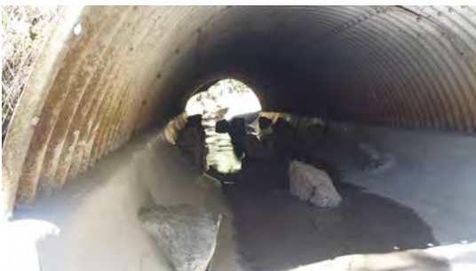
Post-construction - Invert paving and fish rocks installed (9/29/16)
