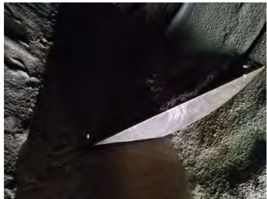
Baffle inside culvert during lower flow – steel corner baffles are bolted to culvert
