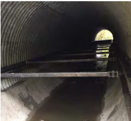
Post-construction bracing and invert paving (10/20/16)
