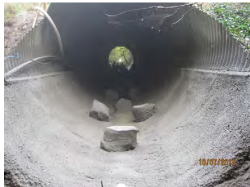
During invert paving - rocks are covered in plastic to keep the concrete off the natural rock surface (10/7/16)
