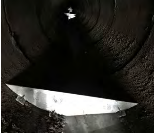
Internal culvert baffles
