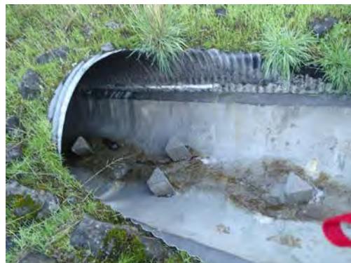
Roughness features creating turbulence, increased water depth, and longer flow path during low flow (10/26/16)
