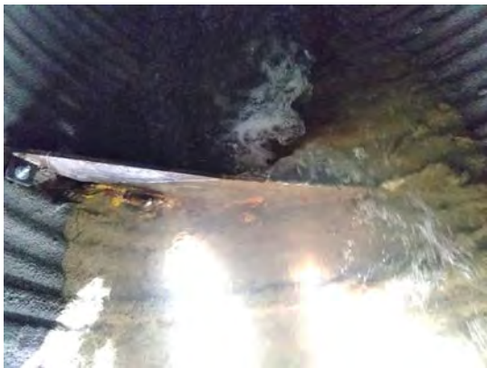
Baffle inside culvert showing resting habitat and deeper water
