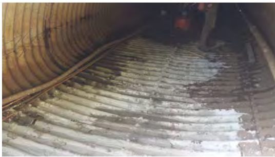
Grouting the invert to fill voids under the invert and reinforce the floor so that the fish rocks and invert paving can be installed (9/21/16)
