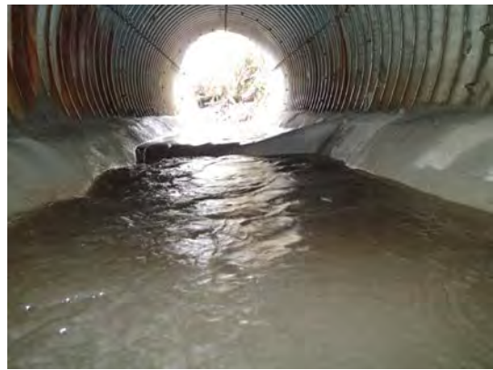
Sloped weir looking upstream toward culvert inlet (10/26/16)
