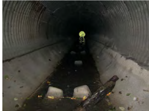
Inside culvert showing invert paving and simulated fish rocks – some debris on double rock installation
