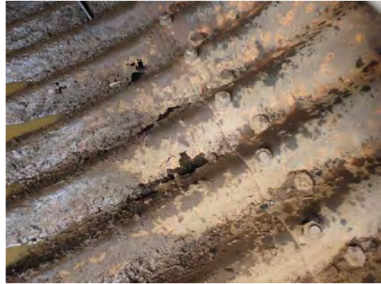
Rusted invert and voids under the culvert (9/20/16)
