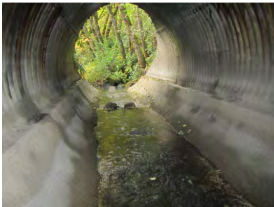
Looking downstream toward culvert outlet showing weir
