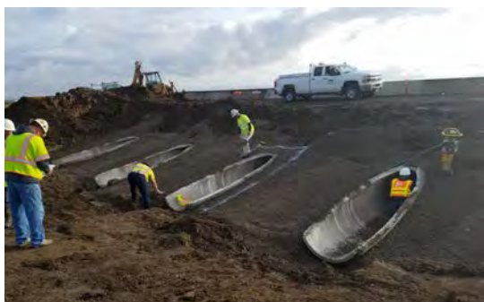
New culvert outlets in construction
