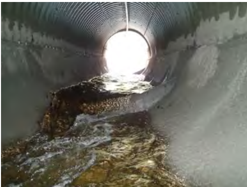
The slump in the middle of the pipe resulted in a less backwater at this weir location (near inlet) than anticipated (10/26/16)
