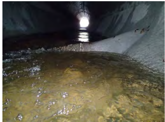
Typical sloped weir configuration with low flow (10/26/16)
