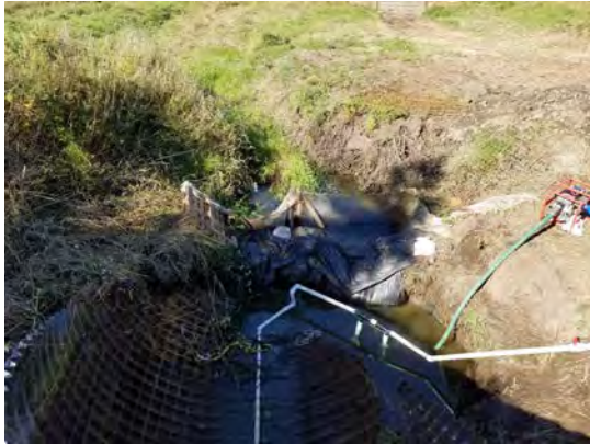
In-water work area isolation at culvert inlet - 2017
