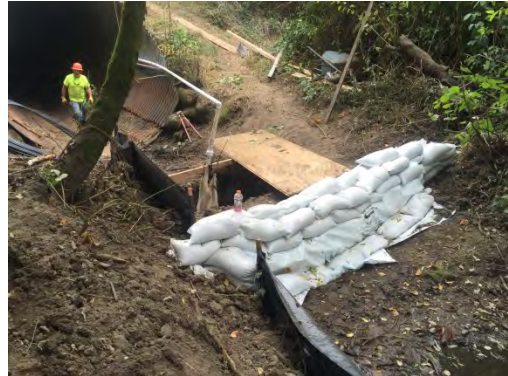
Work area isolation. The stream was not running but there were isolated pools in the channel (10/4/16)
