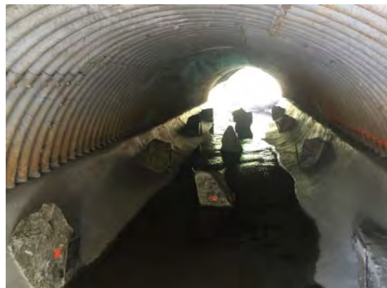
Post-construction - Invert paving and fish rocks installed (9/29/16)
