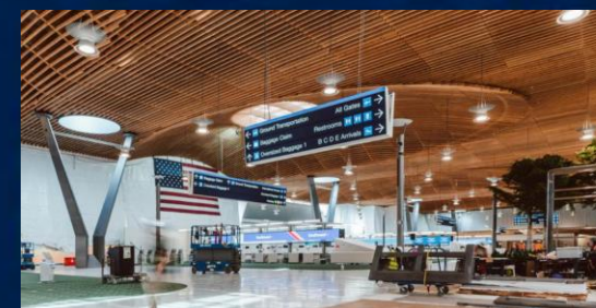
PORTLAND INTERNATIONAL AIRPORT 400,000-square-foot mass timber roof
