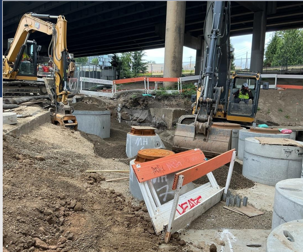
Center: Crews continue manhole and piping work on stormwater facilities
