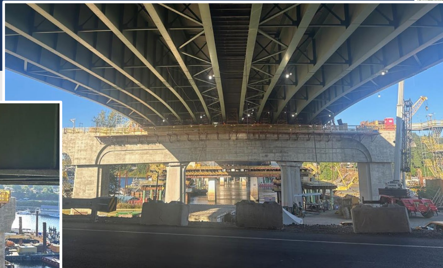
Progress at Pier 3
