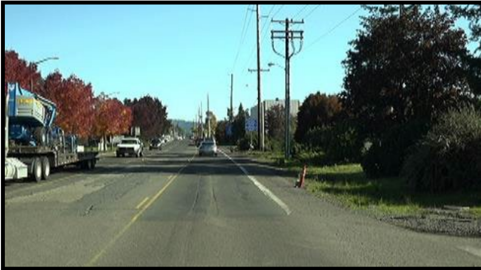
Sidewalk and bike lanes were missing along the road in Dundee, OR before the project.
