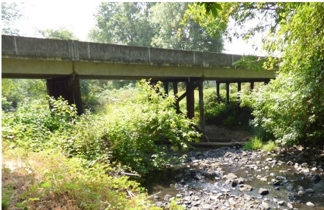
Prior to Construction
