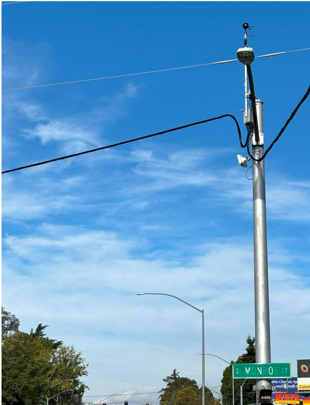
INSTALLED RADAR DETECTION
