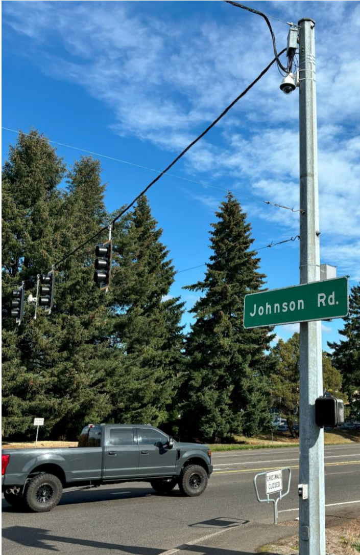
INSTALLED PTZ CAMERA
