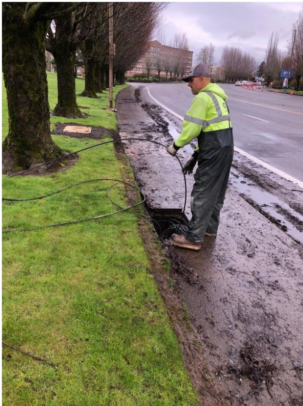
FIBER OPTIC INSTALLATION
