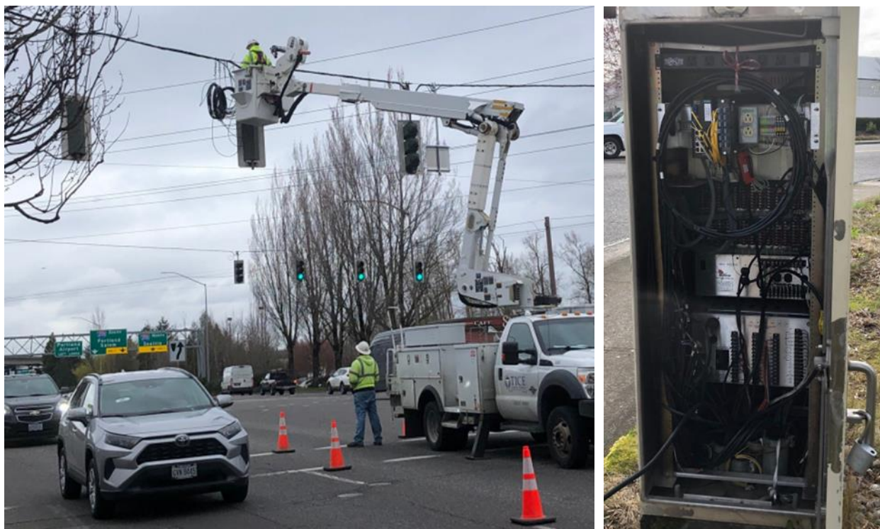
LEFT: INSTALLATION OF FIBER OPTIC CABLE; RIGHT: TRAFFIC SIGNAL CONTROLLER UPGRADES
