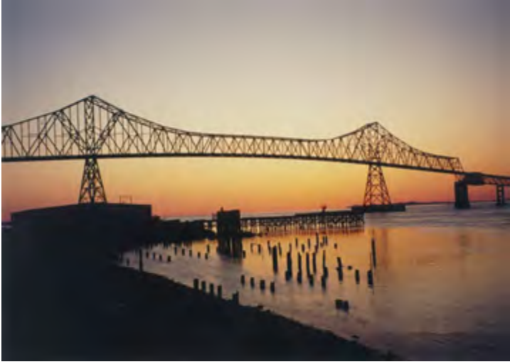
Maintaining a state of good repair is an important prioritization framework for Oregon's bridges and highways.
