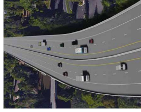
Rendering of retrofitted, widened viaduct cross-section
