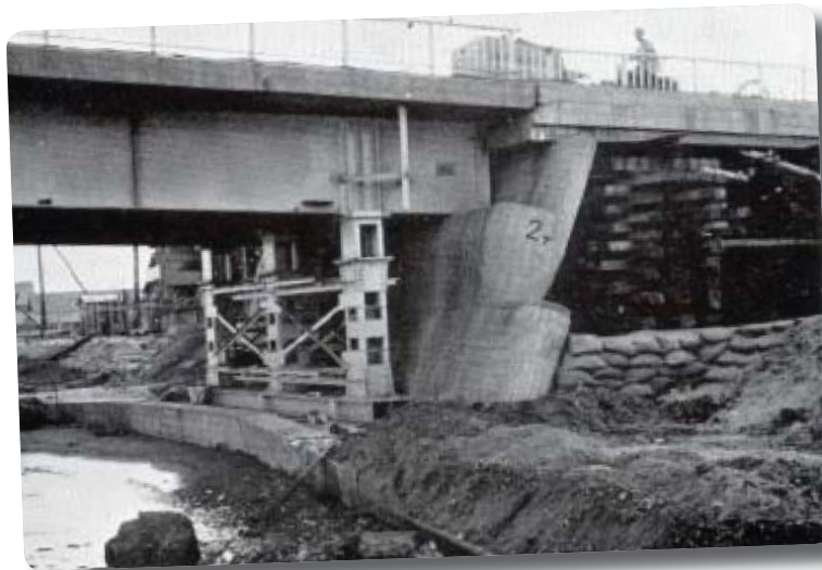
Figure 2.1 : Bridge pier damage resulting from liquefaction and lateral displacement of foundation soils (Yachiyo Bridge, 1964 Niigata, Japan)
