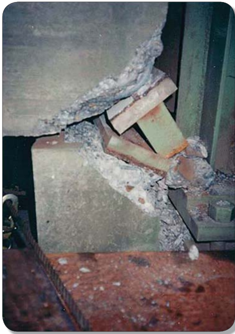
Figure 3.3: Failed Rocker Bearings (Yamhill River Bridge)
