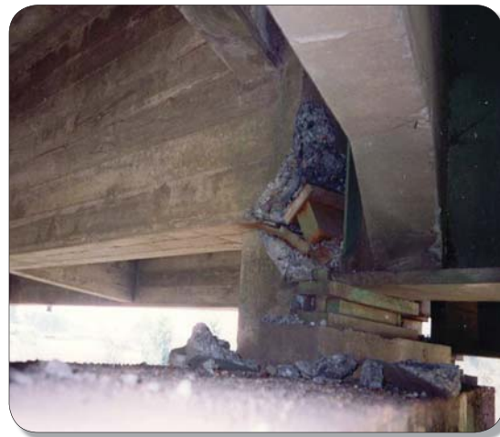
Figure 3.3: Failed Rocker Bearings (Yamhill River Bridge)
