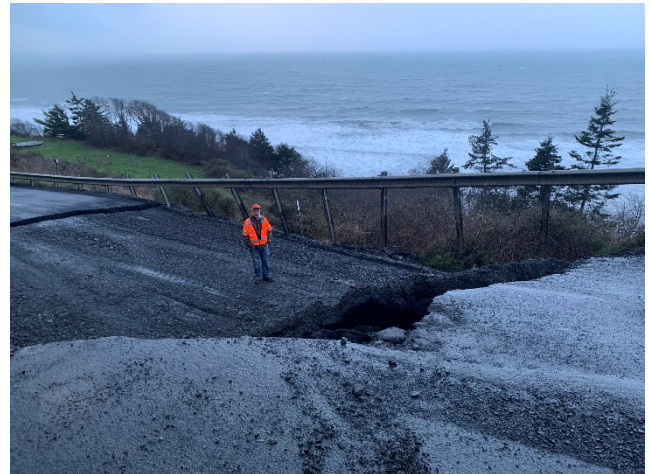
Figure 1: Example of winter deep seated landslide failure and impact to road (Arizona Inn January 2023).
