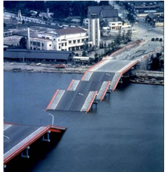
Figure 1: Damage to Showa Bridge in the 1964 Niigata earthquake due to liquefaction-induced lateral spreading (source: NISEE)
