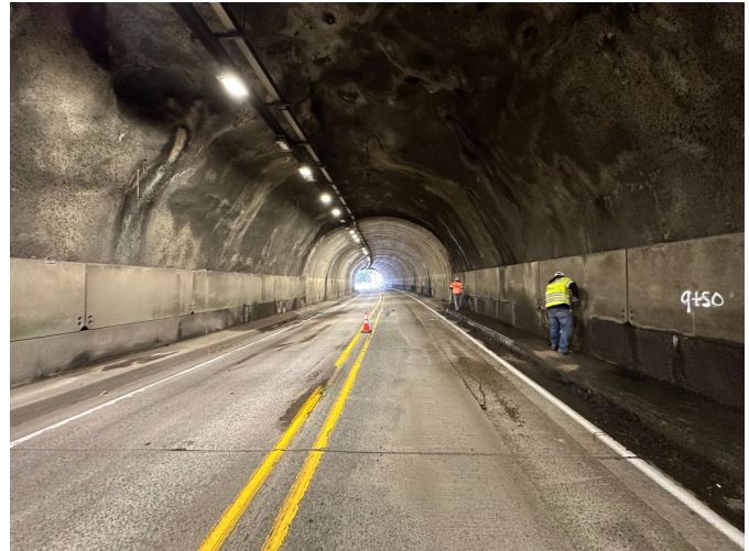
Figure 1: Arch Cape tunnel inspection, both lanes closed
