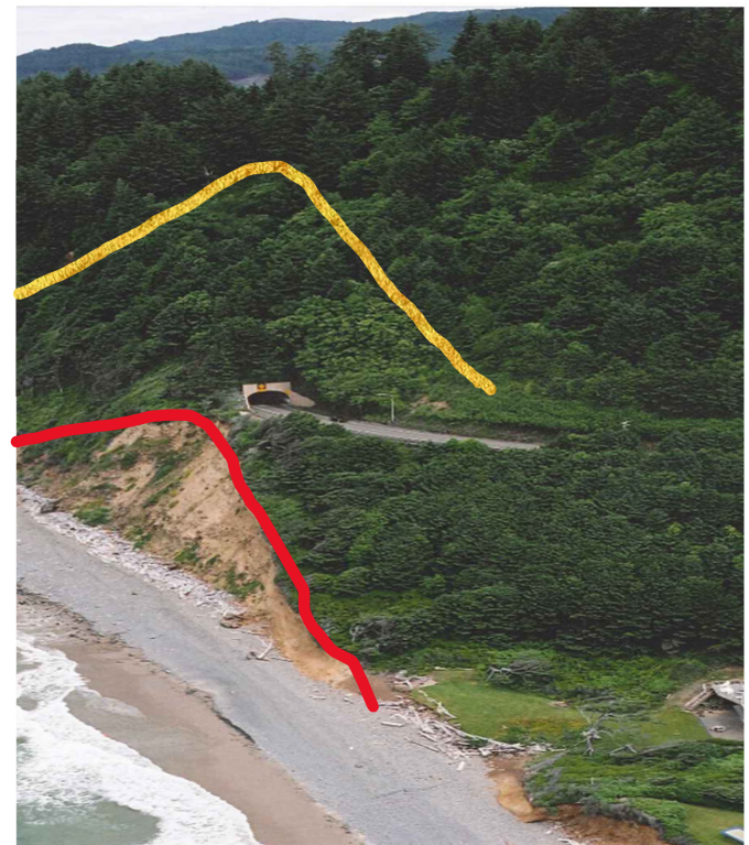
Figure 2: Note the erosion impacts (red) and landslide (yellow) presenting instability risks for the Arch Cape tunnel.
