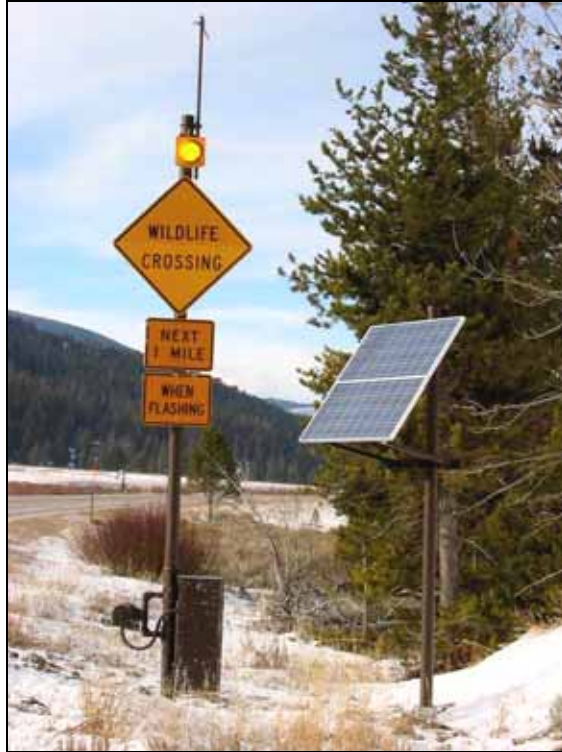
Figure 4.37: Activated warning signal and sign with new text sign “WILDLIFE CROSSING” and solar panel in Yellowstone National Park, Montana, USA (Photo: Marcel Huijser, WTI-MSU)
