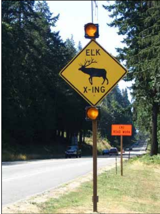
Figure 4.23: Activated warning signal and sign in Sequim, Washington, USA (Photo: Marcel Huijser, WTI-MSU)
