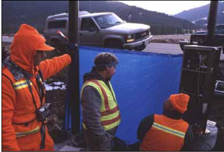
Figure 8.12: STS and MDT representatives at the MT site. After installation the system suffered from a range of technological challenges which required problem identification, problem solving and evaluation (Photo: Marcel Huijser, WTI-MSU).
