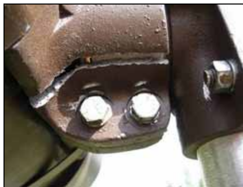
Figure 6.8: The brackets holding the sensors cracked as a result of extreme temperature fluctuations at the MT site (Photo: Marcel Huijser, WTI-MSU)
