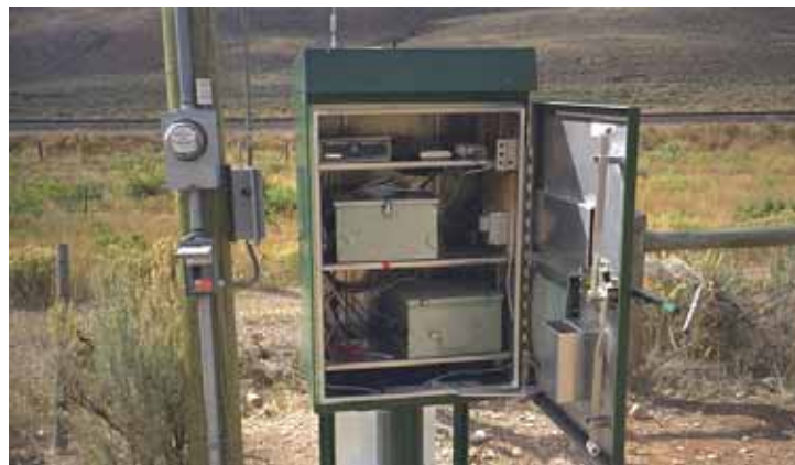
Figure 4.20: Control cabinet at Nugget Canyon, Wyoming, USA. The large boxes are the counters for the animal detections and traffic. The upper shelf holds equipment for downloading data. This equipment used AC power. (Photo: Matt Johnson, WYDOT)
