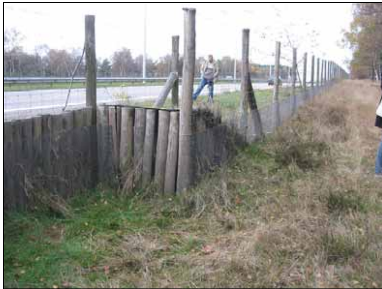
Figure 10.4: Wildlife fences guide large animals towards the crossing area with the animal detection system. Long fence sections should have jump-outs however, to provide an escape for animals that might end up in between the fences in the right-of-way. (Photo: Bethanie Walder)
