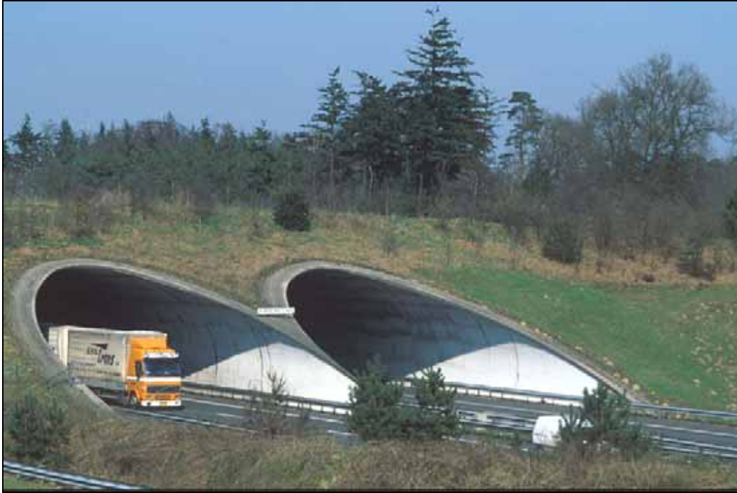
Figure 10.2: Wildlife crossing structures are often combined with wildlife fencing to guide the animals towards the crossing structure. Since some animals may walk the other way and cross the road where the fence ends, an animal detection system may be applied also. (Photo: Marcel Huijser, WTI-MSU)
