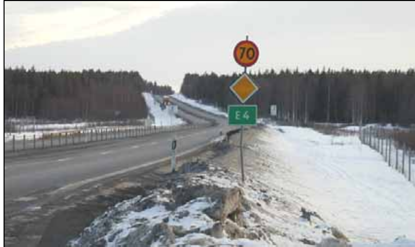
Figure 4.13: The crossing area in Rosvik, Sweden. Note the two lanes one direction and one lane in the other direction separated by a wire fence (Photo: Kjell Ståhl/Road Administration, Luleå)
