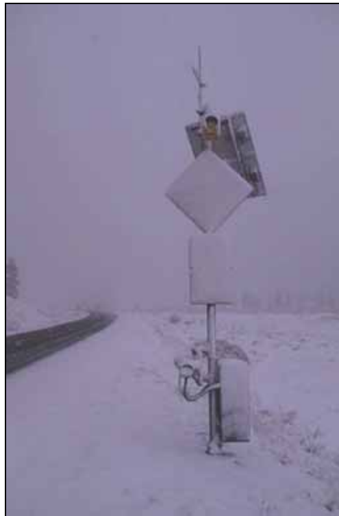
Figure 8.9: Snow may temporarily cover warning signs and signals (Photo: Marcel Huijser, WTI-MSU)
