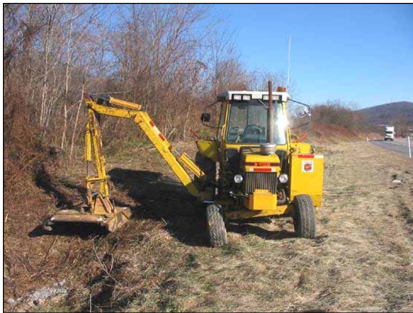
Figure 5.27: Before installation the high shrubs and weeds were cut and branches of trees were removed at the PA site. (Photo: Marcel Huijser, WTI-MSU)
