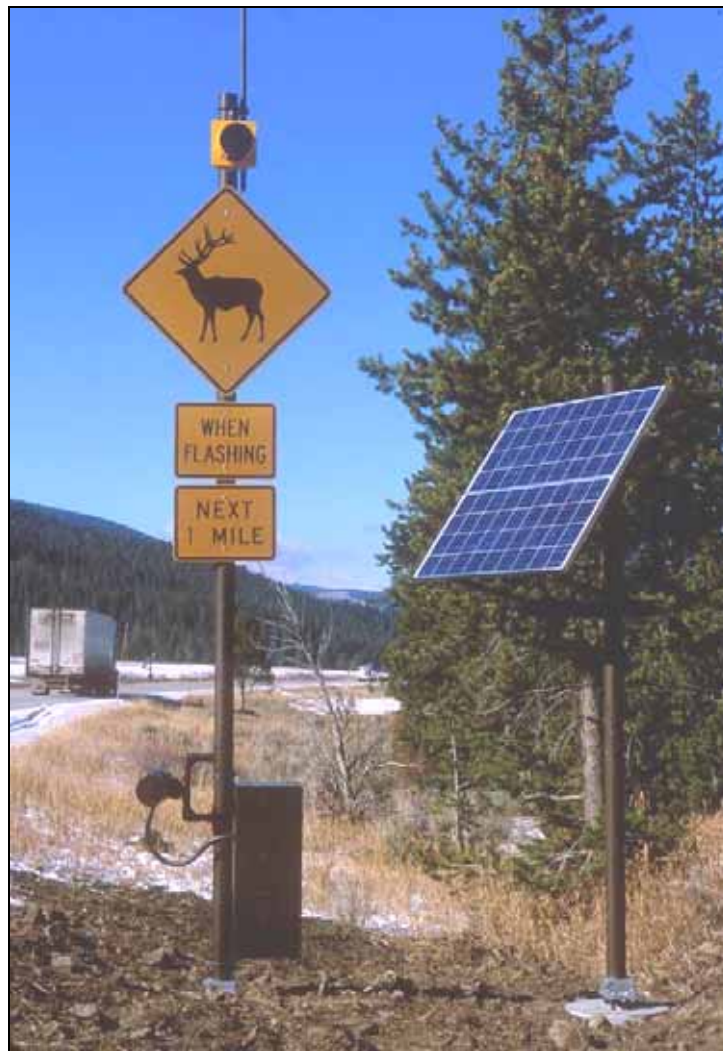
Figure 4.36: Original warning signal and sign in Yellowstone National Park, Montana, USA. A sensor is attached on the left side of the post; a cabinet with circuit boards and batteries is attached to the right side of the post. (Photo: Marcel Huijser, WTI-MSU)
