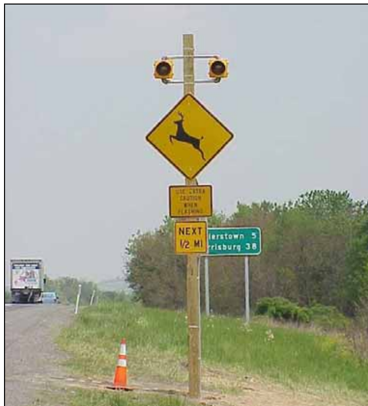
Figure 4.38: Warning signal and sign in Thompsontown, Pennsylvania, USA (Photo: Rhonda Stankavich, PENNDOT)
