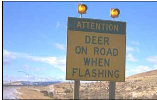
Figure 4.15: Activated warning signals and sign at Nugget Canyon, Wyoming, USA (Photo: Bill Gribble/WYDOT)
