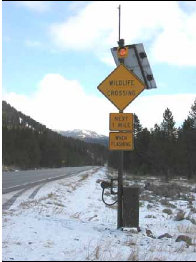
Figure 5.10: Activated warning signal, text sign “wildlife crossing” and solar panel at the MT site (Photo: Marcel Huijser, WTI-MSU)
