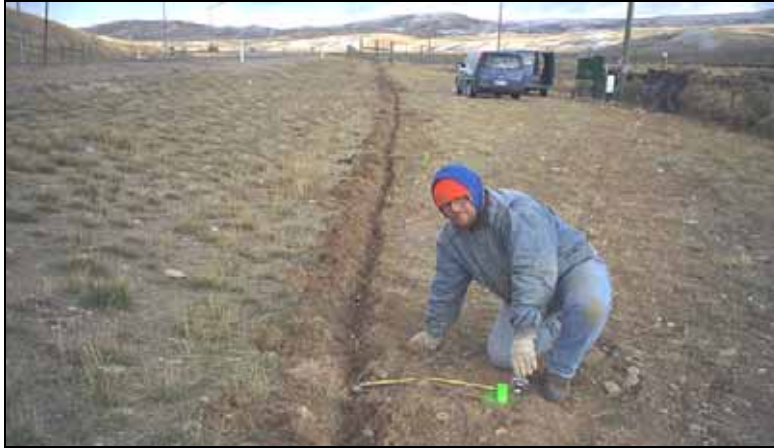
Figure 4.17: Re-installation of the geophone system at Nugget Canyon, Wyoming, USA. The sensors were approximately 10 m (33 ft) apart at a depth of about 10 cm (4 in) below ground level to the top of the sensor. (Photo: Bill Gribble/WYDOT)
