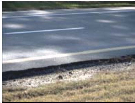
Figure 5.31: Eliminate shoulder drop-off or provide wedge
