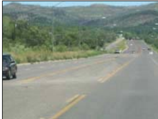
Figure 3.6: Two-way left-turn lane
