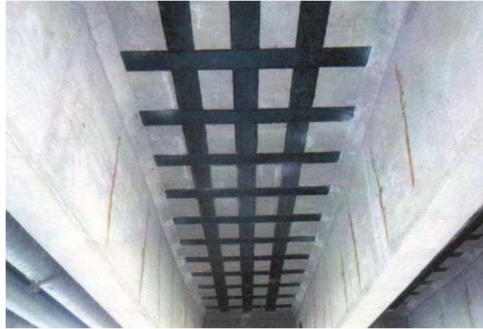
Figure 2.3: Strengthening of concrete bridge deck
