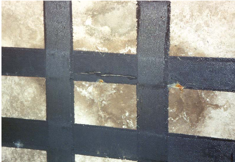
Figure 7.A5.10: Split in composite
