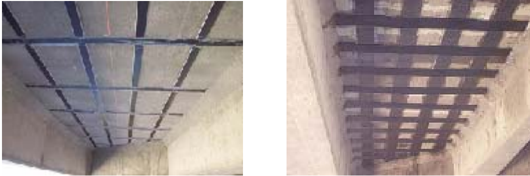
Figure 9.1: Onsite rehabilitation of bridge deck
