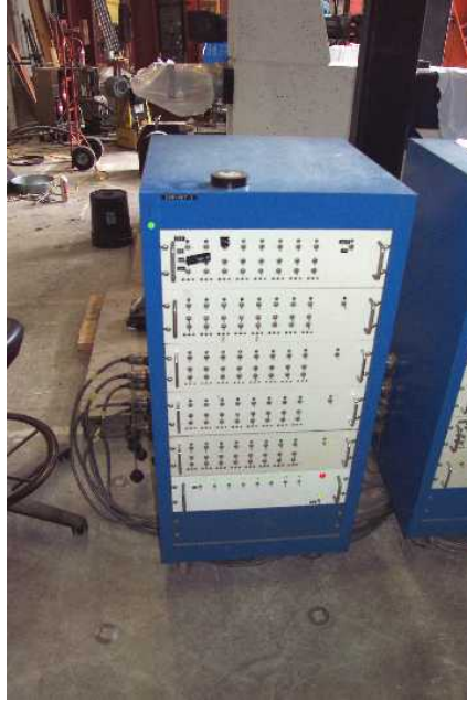
Figure 4.59: Multi-channel data acquisition bay
