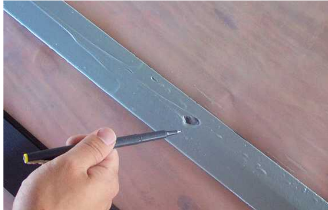
Figure 2.36: Formation of void during putty application
