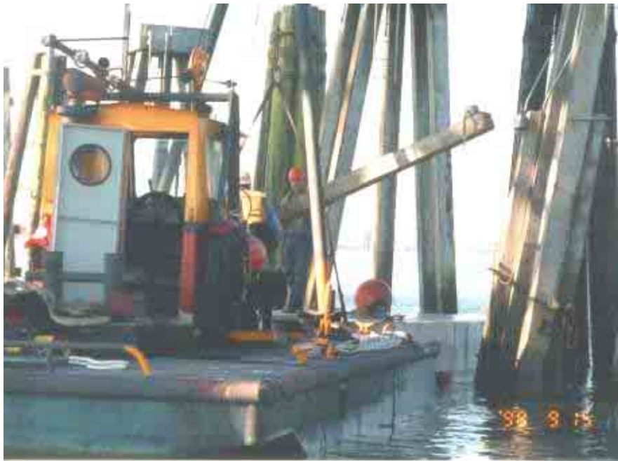
Figure 4.1: The Test Beam being Lifted onto the Barge.
