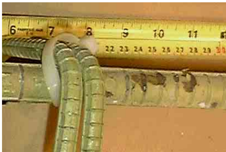
Figure 4.15: Observed Corrosion of Longitudinal Rebar in the Submerged Zone
