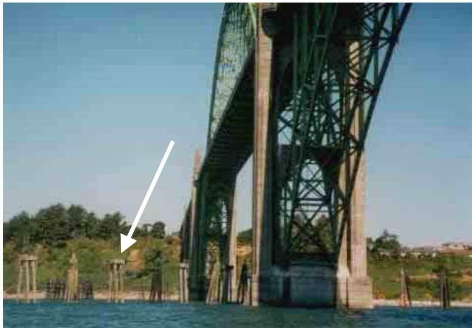
Figure 1.2: Overall View Showing Concrete Dolphins in Yaquina Bay
