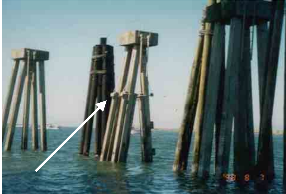
Figure 1.3: Concrete Beams Attached to the Dolphin in the Middle of the Picture
