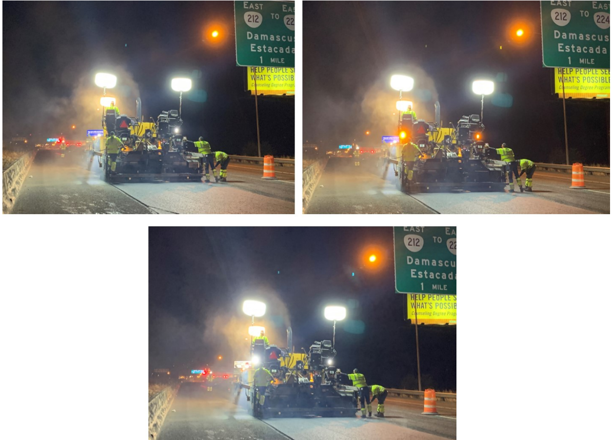
Figure 3.3: Only balloon lights on (top-left), amber lights on (top-right), and white lights on (bottom) (case study 2)
