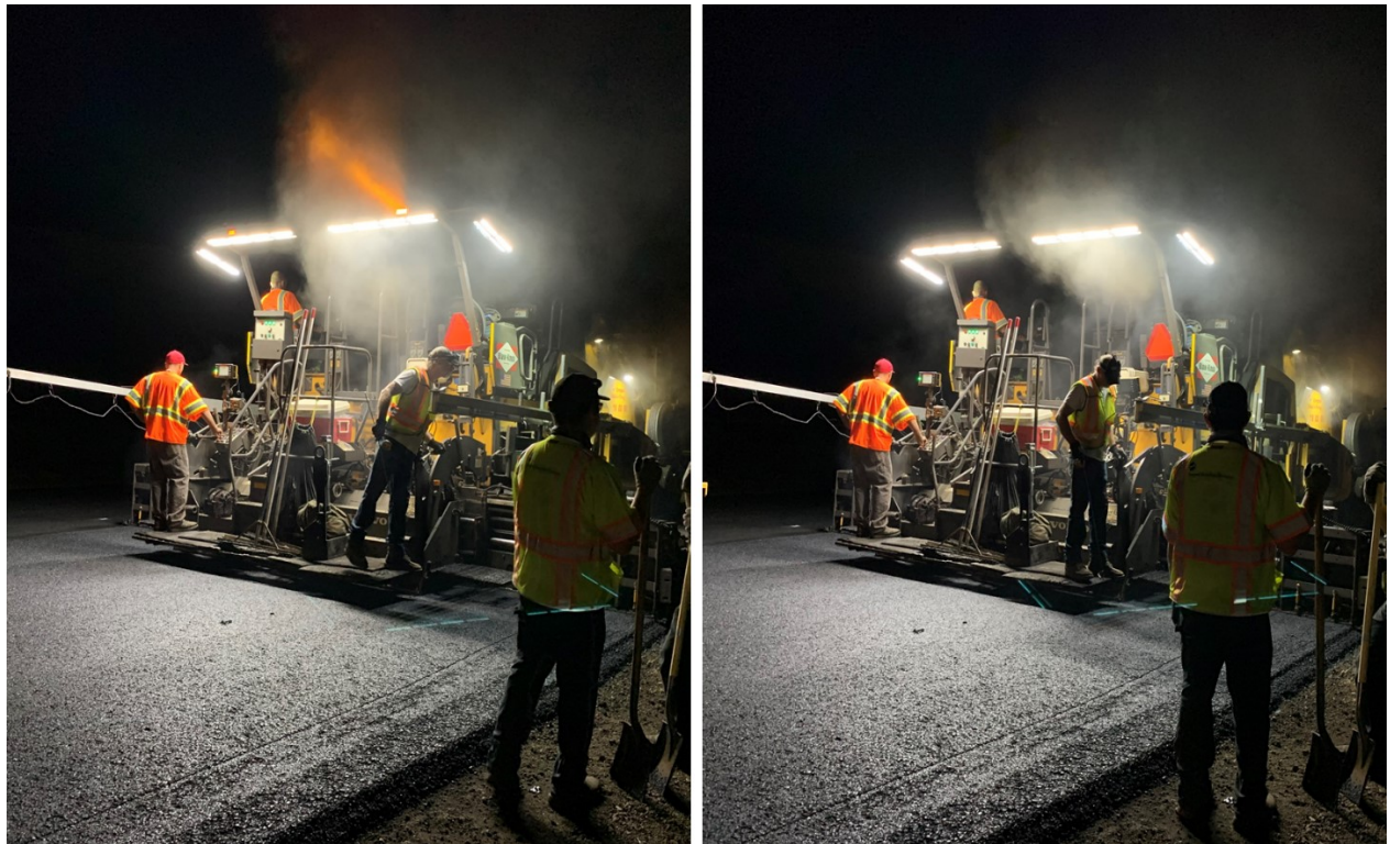
Figure 3.1: Paver with flashing amber lights on (left) and amber lights off (right) (case studies 1 and 3)
