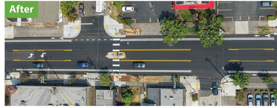
Above: North Lombard Street between North Drummond Avenue and North Oatman Avenue after safety improvements.
