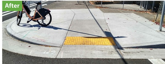
Above: Upgraded ADA accessible sidewalk curb ramps for greater safety for all users after improvements.
