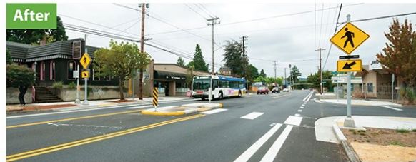
Above: A RRFB and median refuge island for safer and more visible pedestrian crossings after improvements.
