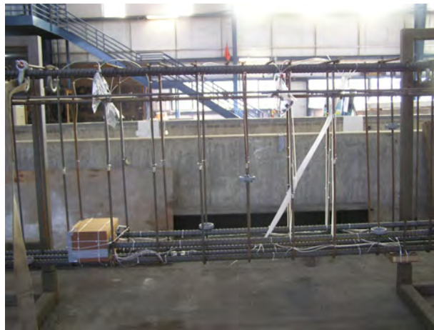
Figure 3.10: Example of specimen geometry prior to concrete placement
