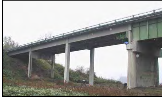
Figure B.1: South approach spans of Willamette River Bridge on OR 219 (Higgins, et al. 2004)
