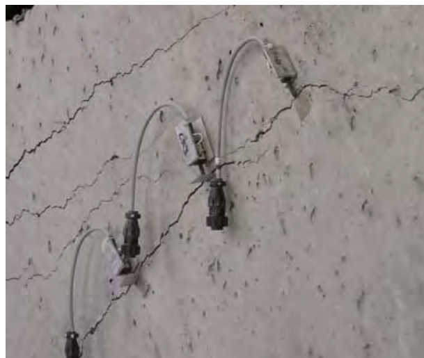
Figure 3.22: Typical crack width sensors
