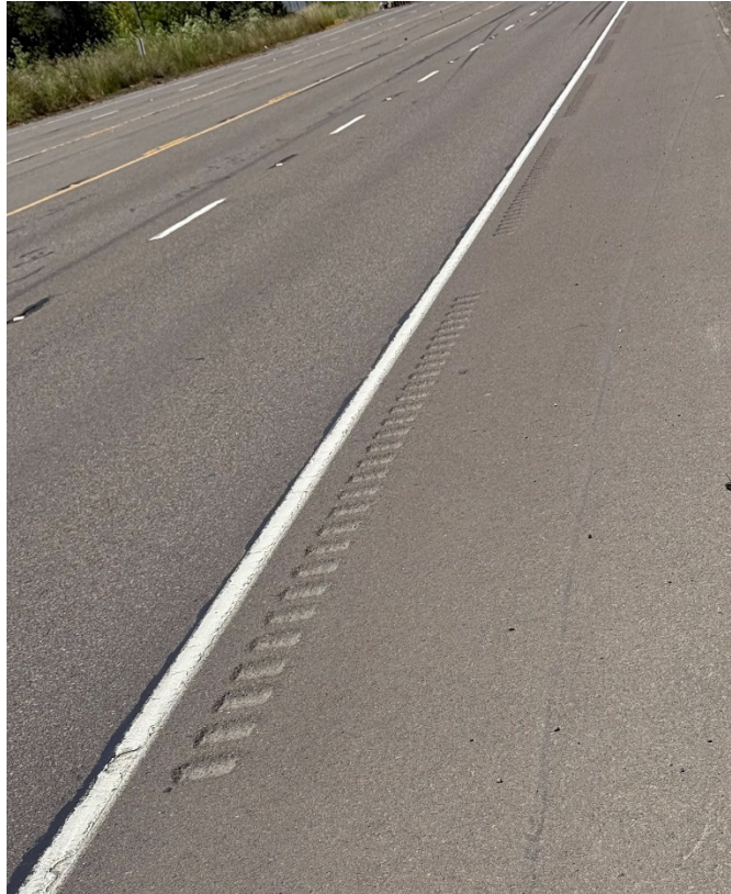
Figure 1-2: Shoulder Rumble Strip on Corvallis-Lebanon Hwy 210, Albany, OR
