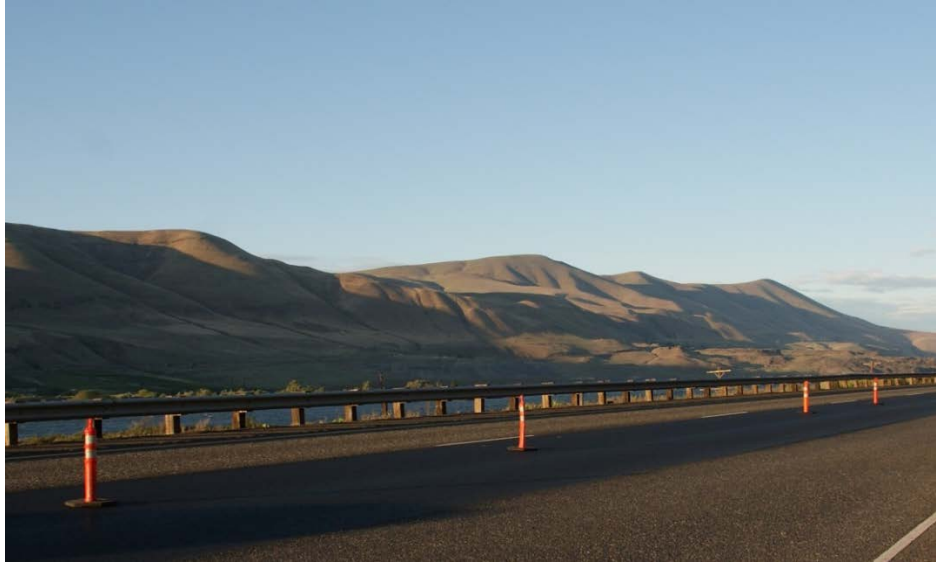
Figure 2.2: Tubular Markers on Roadway
