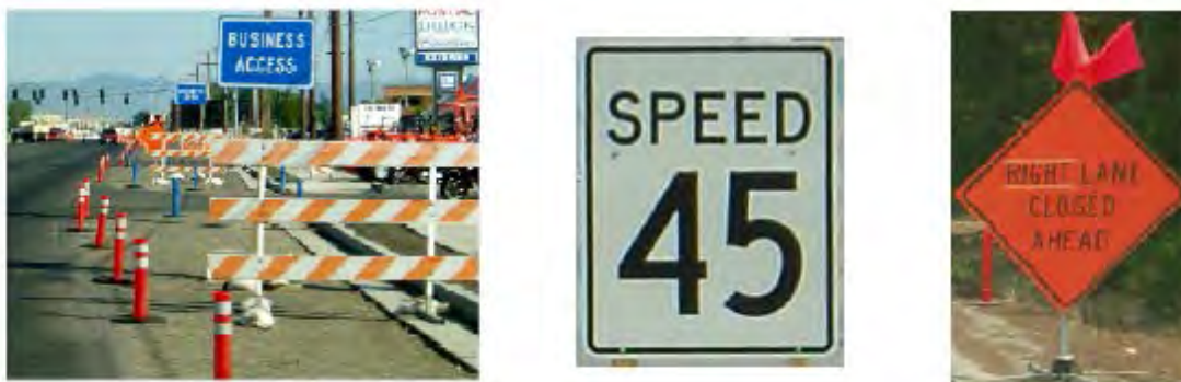
Figure 2.5: Examples of Temporary Signs (ODOT 2014)
