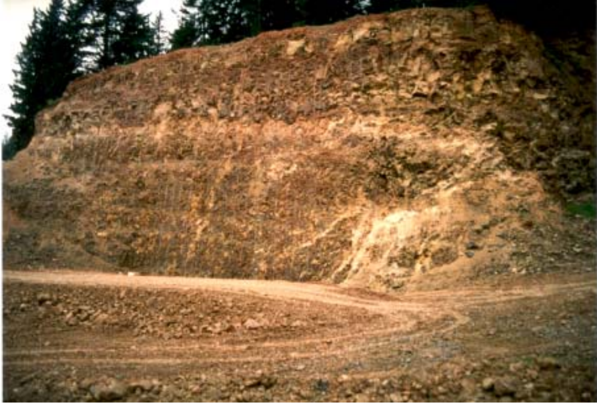
Figure 3.2: 24.4-meter high, 4V:1H presplit slope (Oregon test site)
