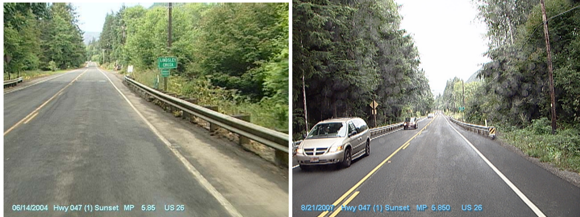
Figure 5.48: Conditions in 2004 (before) and in 2007 (after) showing the upgraded guardrail at Lindsley Creek BR 03095, MP 5.85
