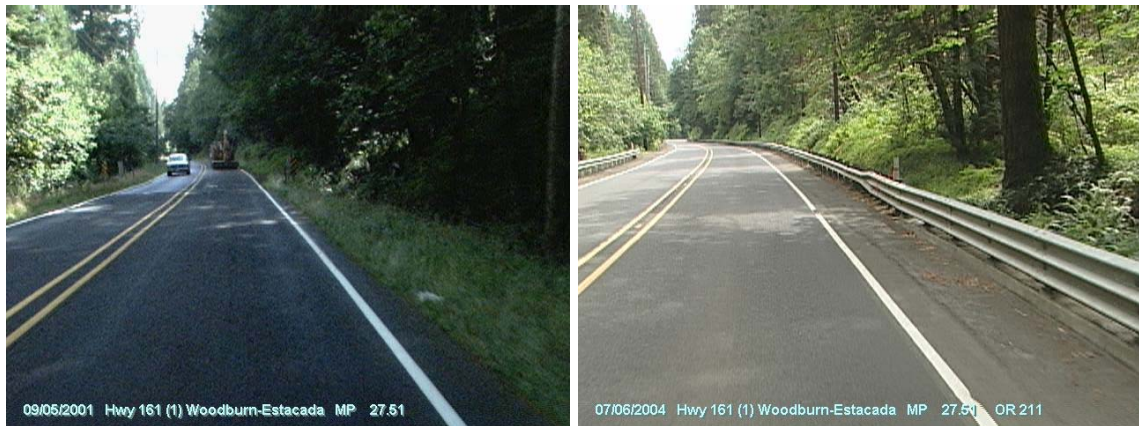
Figure 5.30: Conditions in 2001 (before) and in 2004 (after) showing the added guardrail/upgraded culvert at Little Cedar Creek (MP 27.51)
