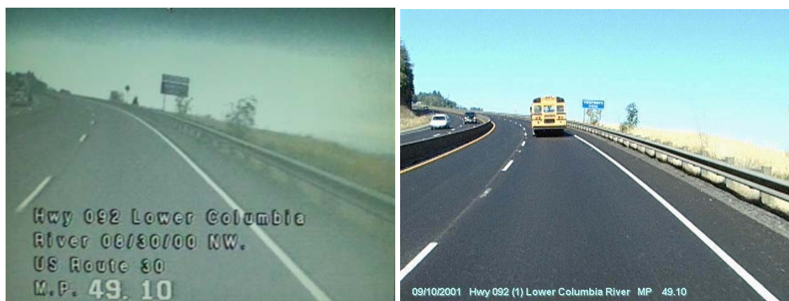
Figure 5.8: Conditions in 2000 (before) and 2006 (after) showing guardrail and pavement markings at MP 49.10
