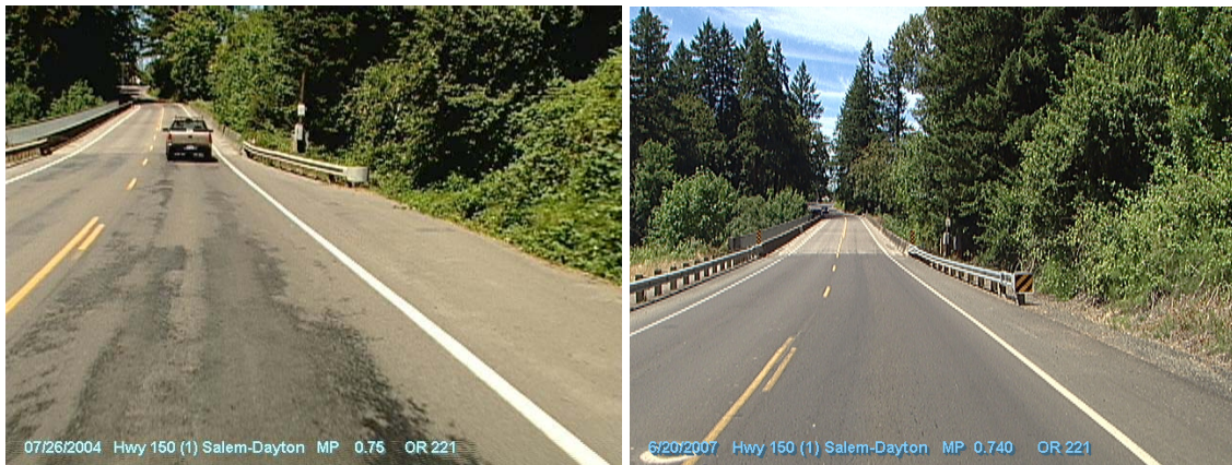
Figure 5.44: Conditions in 2004 (before) and in 2007 (after) showing the upgraded guardrail ends at MP 0.75
