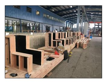
Figure 3.16: Formwork construction
