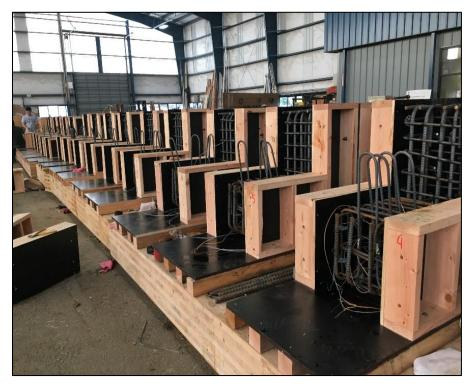
Figure 3.18: Cage is inserted into formwork
