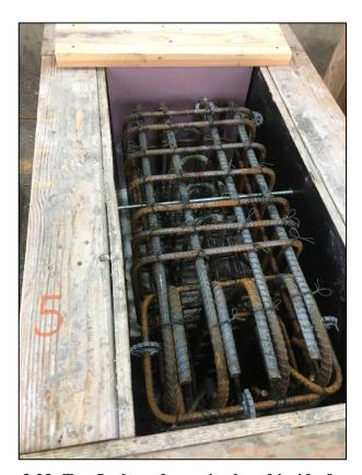
Figure 3.23: Top L-shaped cage is placed inside formwork
