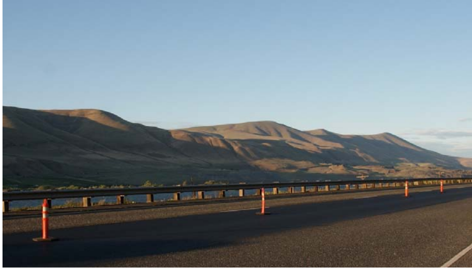
Figure 2.2: Tubular Markers on Roadway
