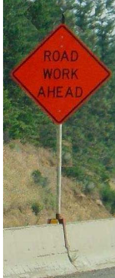
Figure 2.7: Concrete Barrier Sign Support (ODOT 2011)
