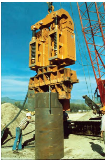
Figure 2.7 Use of (a) oscillator rig, (b) vibro-hammer, and (c) twister bar to advance casing (after Brown et al. 2010)
