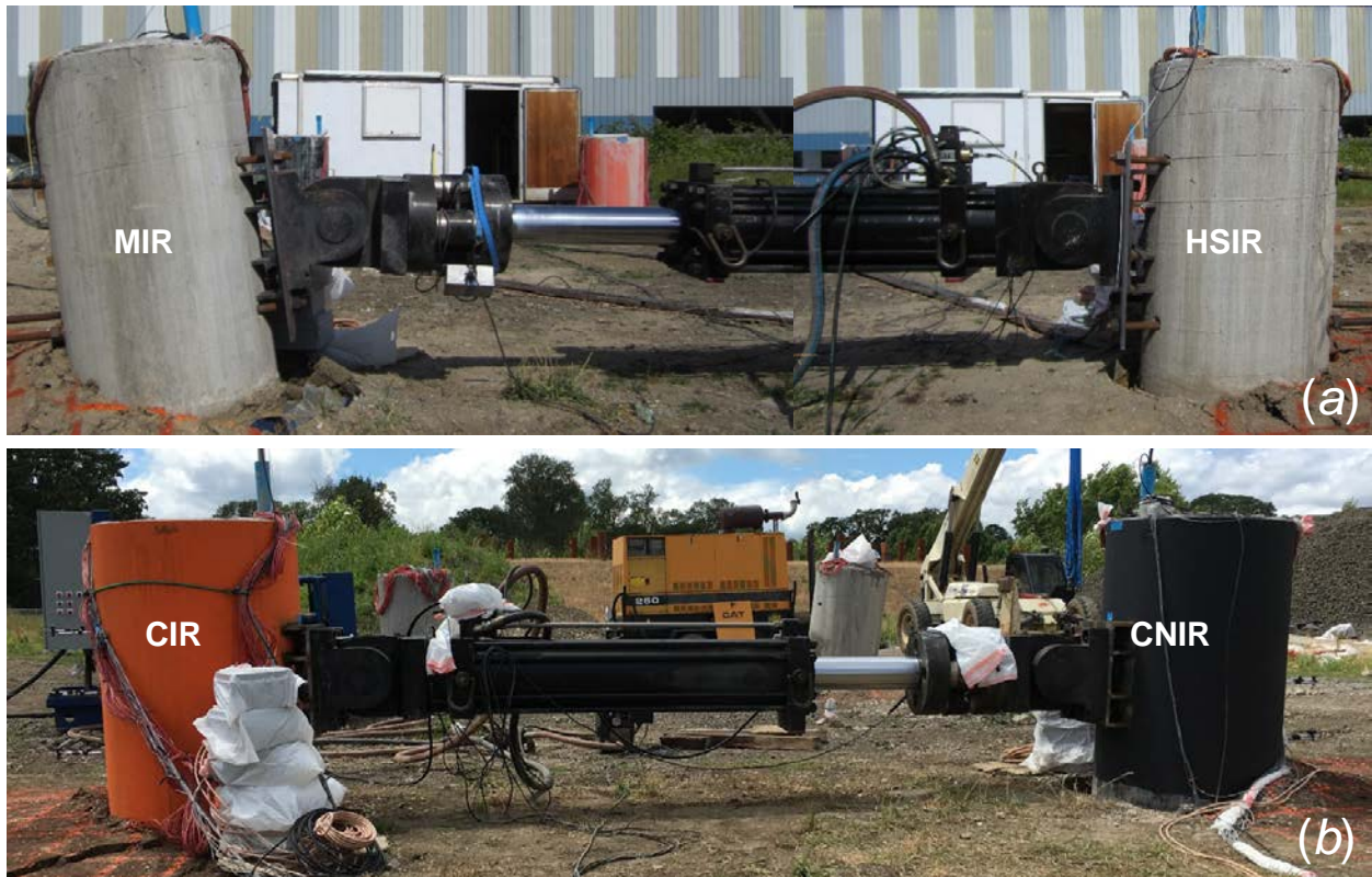
Figure 5.13: Lateral loading tests setup for (a) uncased shafts and (b) cased shafts. Note, the photos were taken at the applied displacement of 447, 206, 213, and 205 mm (17.6, 8.11, 8.39, and 8.07 in) for MIR, HSIR, CIR, and CNIR, respectively.
