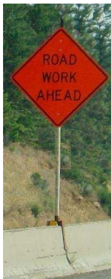
Figure 2.7: Concrete Barrier Sign Support ( ODOT 2011 )
