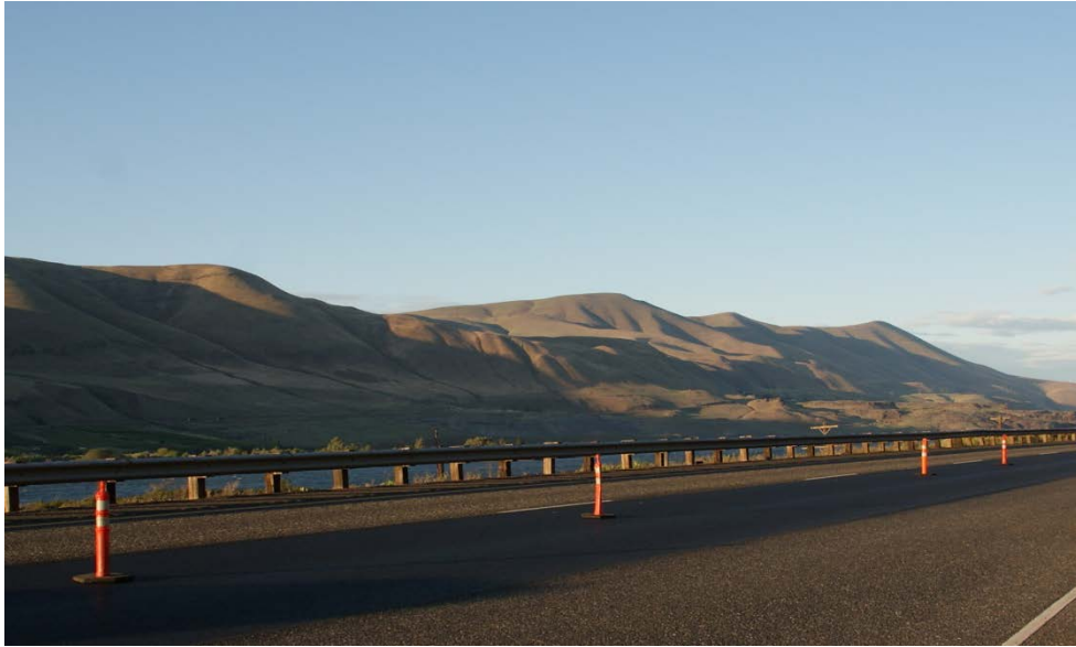
Figure 2.2: Tubular Markers on Roadway
