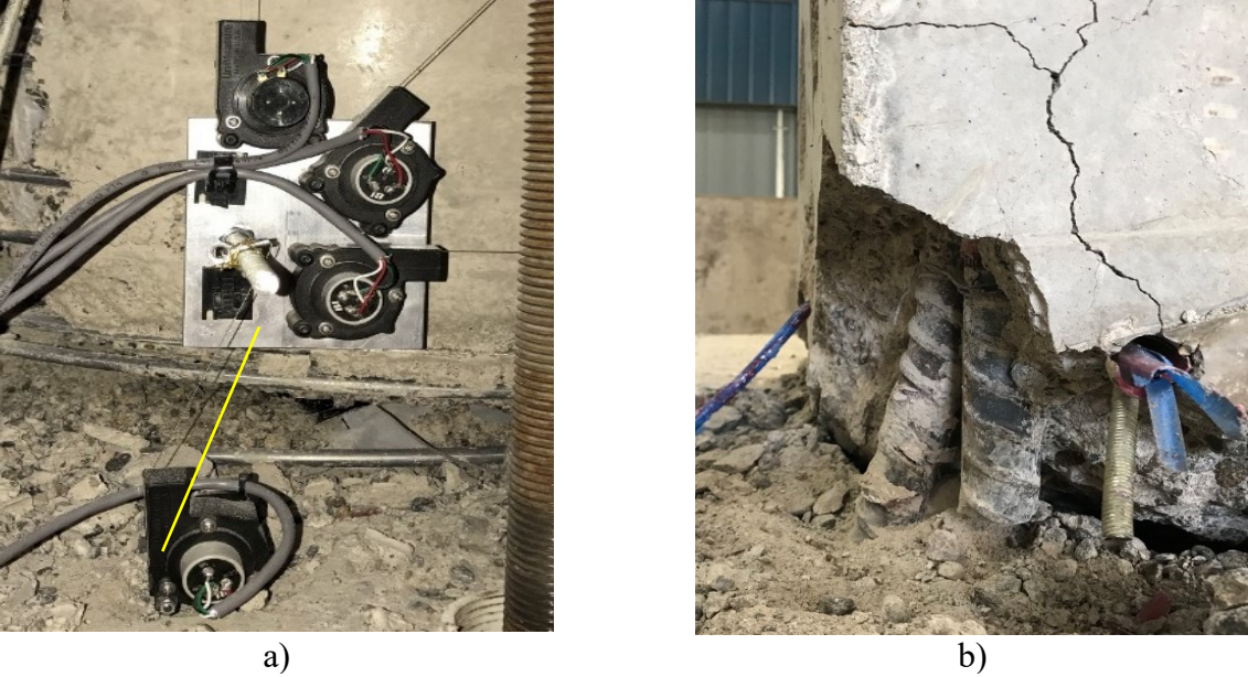
Figure 4.14: Specimen R-S-R-0: a) String Pot showing the sliding of the column at column-footing interface (string highlighted in yellow), b) NW starter bar bent towards South after testing
