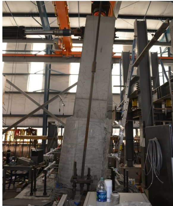
Figure 4.32: Condition of specimen RS-T-R-LTi-90 at peak drift (8.2% drift)
