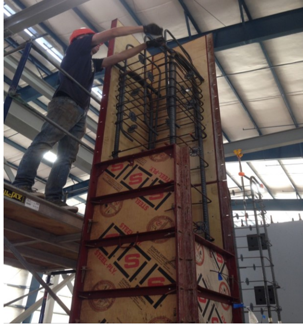
Figure 3.22: Additional reinforcing steel near column loading point for tall columns
