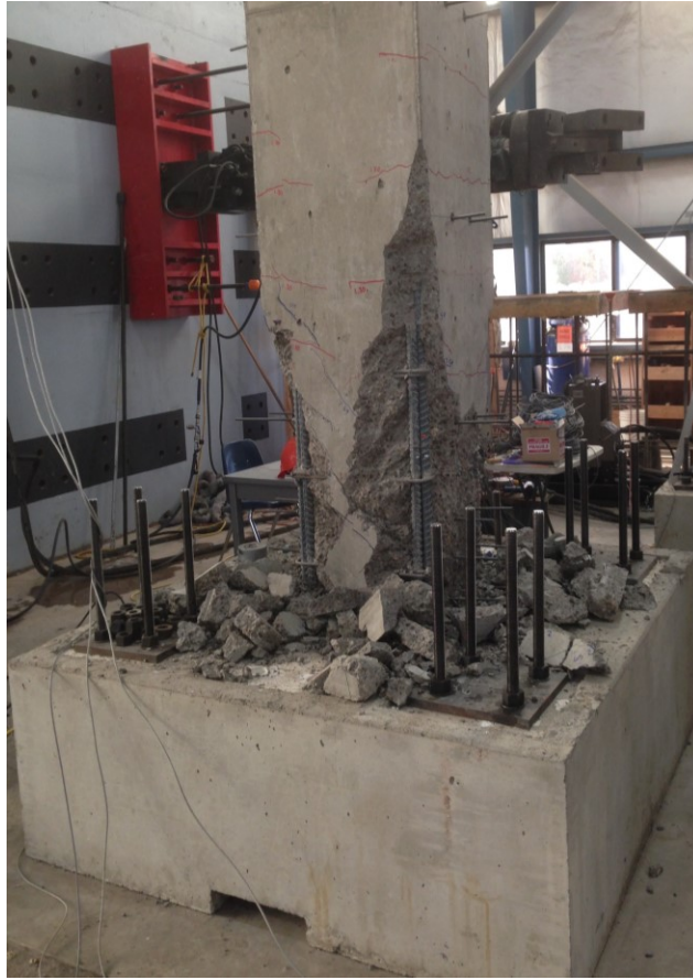
Figure 4.27: Condition of specimen C-T-R at end of test (maximum 5.4% drift)
