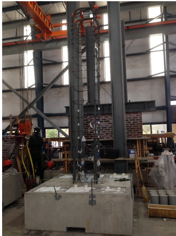
Figure 3.23: Typical reinforcing steel cage for tall column specimens
