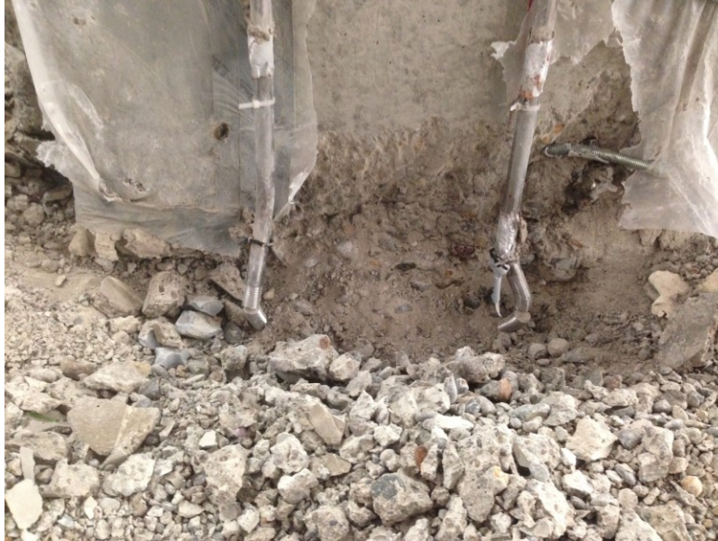
Figure 4.34: Specimen RN-T-R-LTi-90: Fractured SE and SW TiABs ligaments and damage to top of footing (shell removed after testing)
