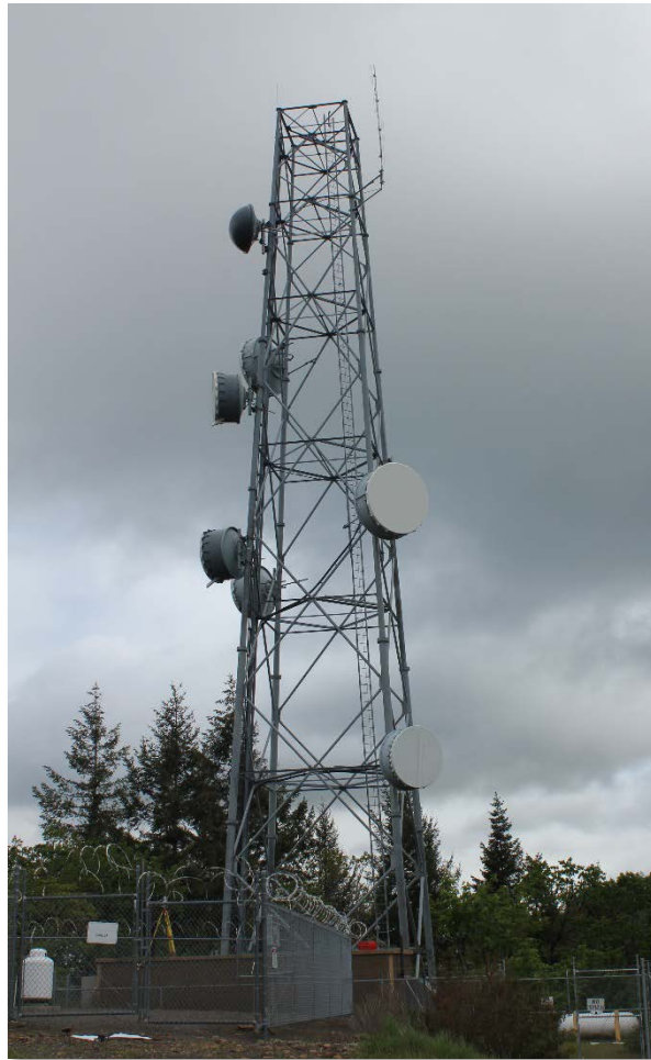
Figure 4.94: Washburn Butte ODOT Communication Tower
