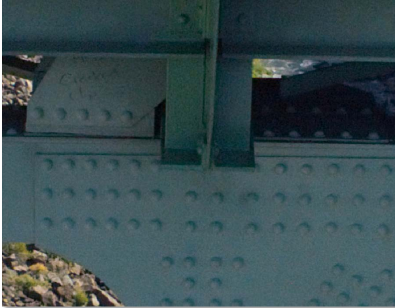
Figure 4.14: Crooked River Bridge bearing connection. (Cropped image)
