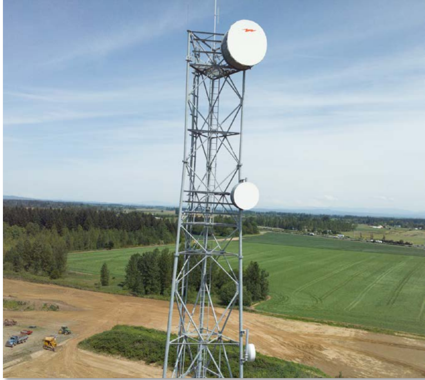
Figure 4.87: Various antenna mounted on Woodburn Tower. Taken with senseFly albris (Full image)
