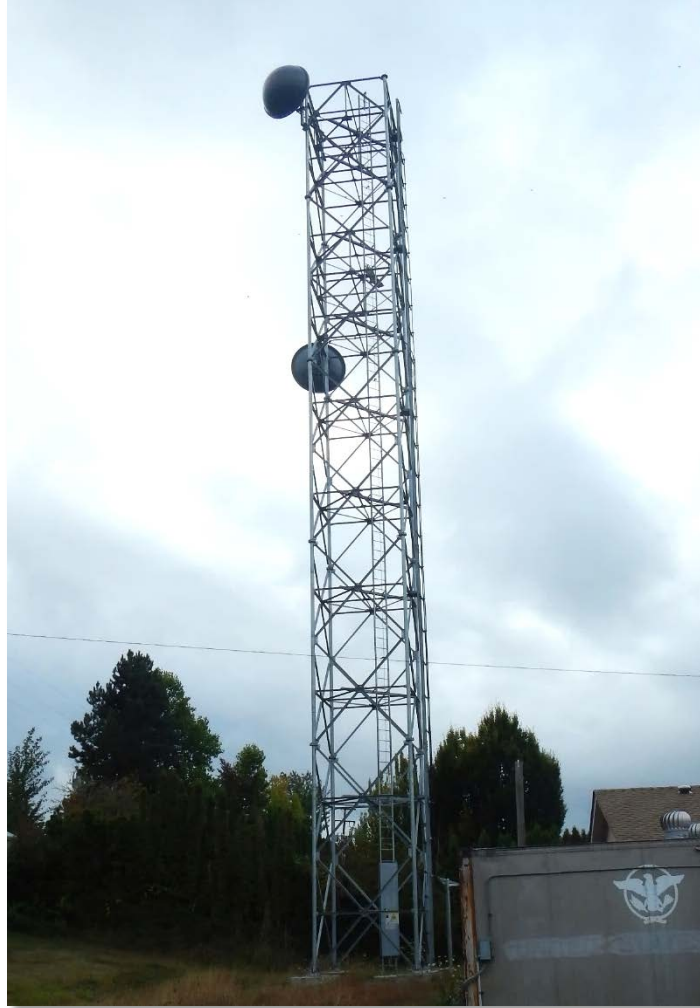
Figure 4.104: Corvallis Maintenance Tower
