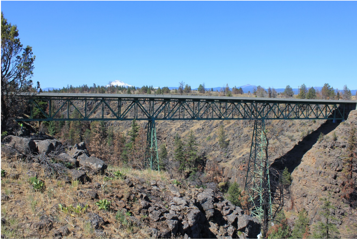
Figure 4.23: Mill Creek Bridge on US 26 in Wasco County, Oregon
