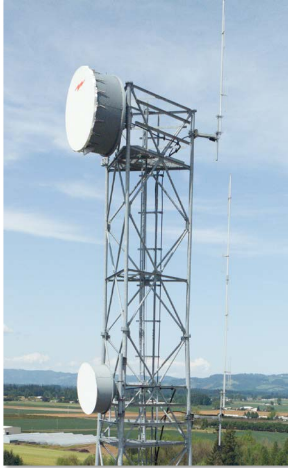
Figure 4.88: Top of Woodburn Tower. Taken with senseFly albris (Full image)
