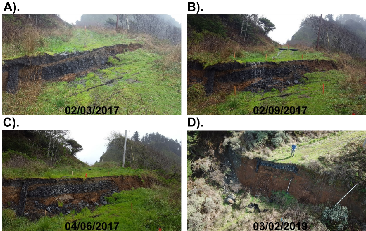
Figure 3.6: Development of a headscarp of a smaller progressive landslide within the main landslide body at Arizona Inn directly above the sea cliff from February 2017 (A) to March 2019 (D).
