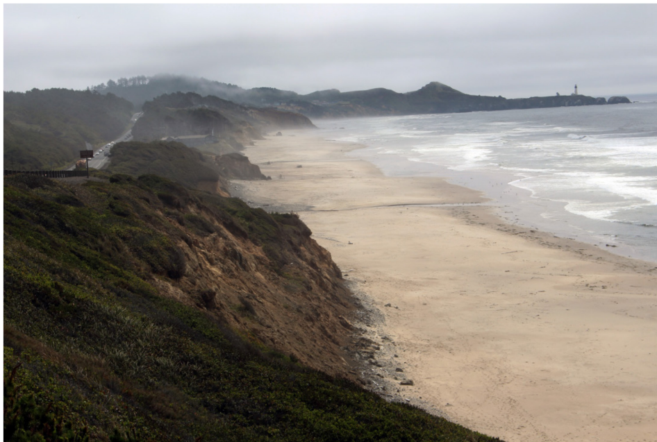
Figure 3.7: Photograph of the Spencer Creek site, facing south, with Highway 101 on the left separated from ocean by the crumbling coastal sea cliff (Near MP 134, August 2016).
