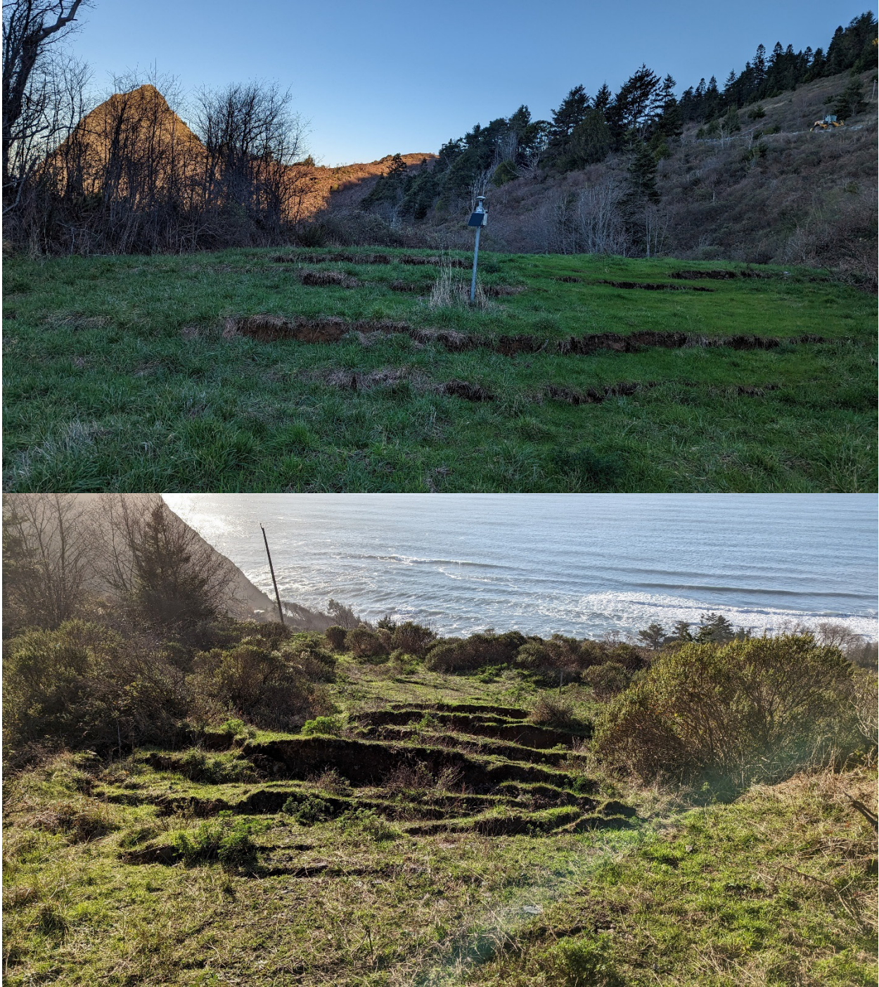
Figure 12.4: Examples of tension cracks (a) near Rover 1 and the cistern and (b) on the upper slopes above the highway. (January 20, 2023)
