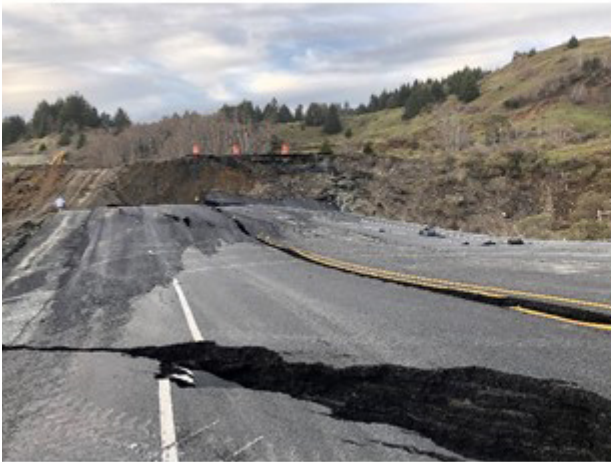
Figure 11.2: Photographs acquired in early March 2019 shortly after the Hooskanaden landslide event. A). Uplift of the beach at the toe of the landslide. B). Overview of the damage caused to Highway 101. C). Close up damage caused to the road by the landslide. D). An example tension crack/scarp from the upper portion of the landslide (above the road).
