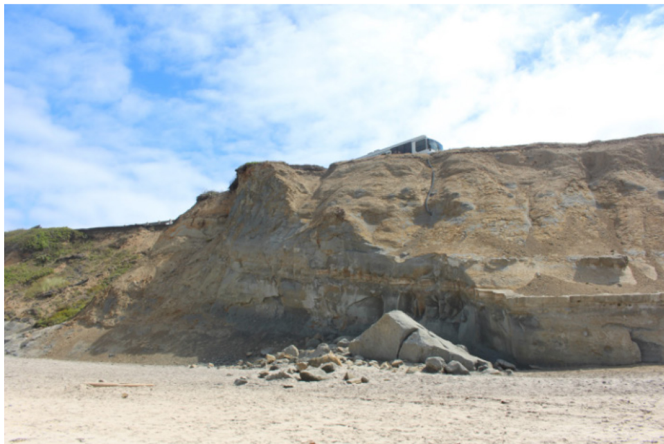
Figure 3.9: Example coastal sea cliff failure at Spencer Creek (facing east, near MP 134, August 2016).
