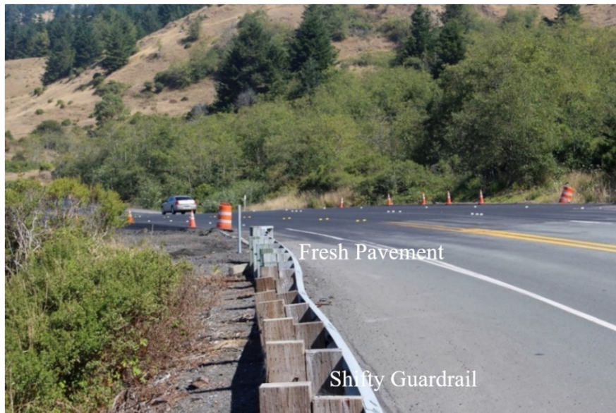
Figure 1.1: Example Evidence of damage to Highway 101 at the Hooskanaden Slide requiring routine repaving of the road (MP344, August 2016).
