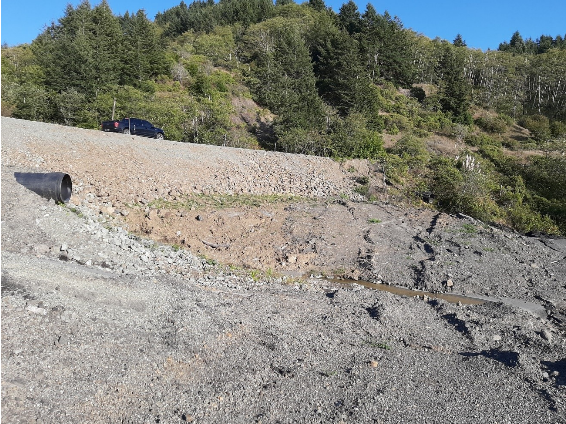
Figure 4.4: Image showing continuous drainage from a culvert installed beneath the newly reconstructed section of US Highway 101, taken in the late summer of 2019.
