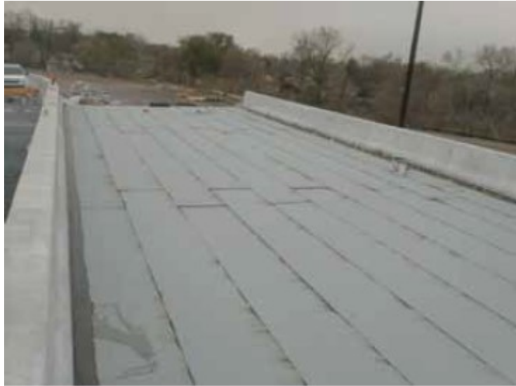
Figure 2.26: Waterproofing roll-on sheet membrane seams (Russell, 2012)
