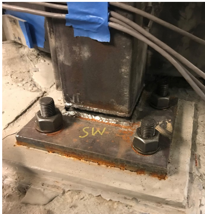
Figure 5.4: Hold-down weld failure
