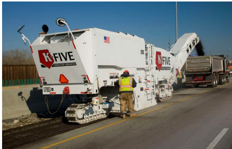
Figure 2.7: Pavement milling operations in the field (West 2010).
