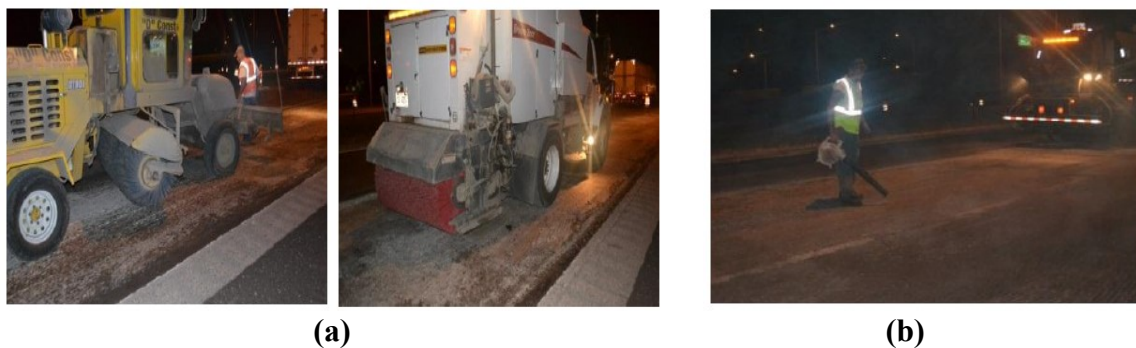
Figure 2.10: Cleaning methods (a) Sweeping and vacuuming and (b) air blasting (Al-Qadi 2012b).
