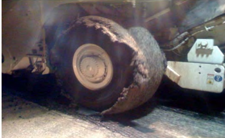
Figure 4.3: Tracking on paver wheels due to excess dust (Mohammad et al. 2012).
