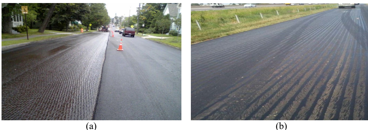
Figure 2.9: Tack coat application uniformity (a) Acceptable tack coat application uniformity (uniform), and (b) unacceptable tack coat application uniformity (non-uniform).
