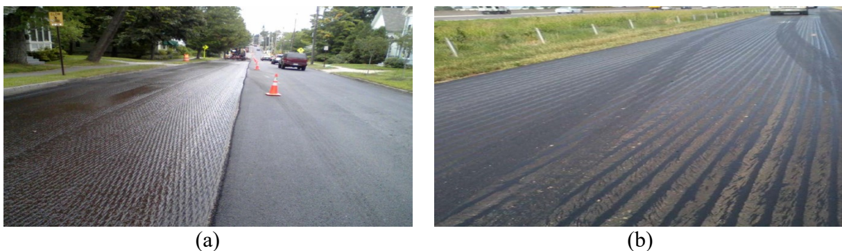
Figure 4.4: Tack coat application uniformity: (a) Acceptable tack coat application uniformity, and (b) unacceptable tack coat application uniformity (streaking) (FHWA 2016).
