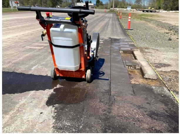
(h) Diamond blade walk-behind saw
