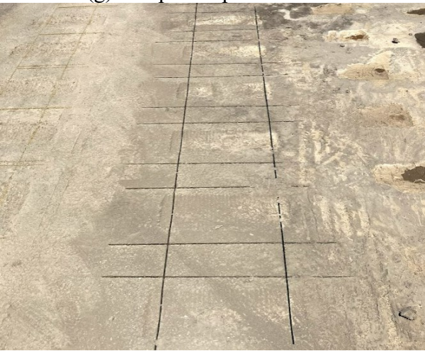
(i) Typical asphalt slab cuts using the walk-behind saw
