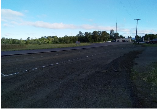
(a) Section before construction (6/25/2020 – 7am)
