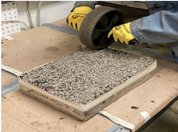
(e) Compacting aggregates
