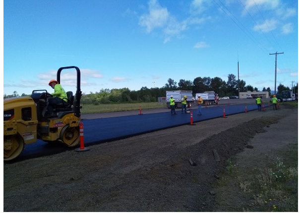
(b) Section construction (6/25/2020 – 12pm)
