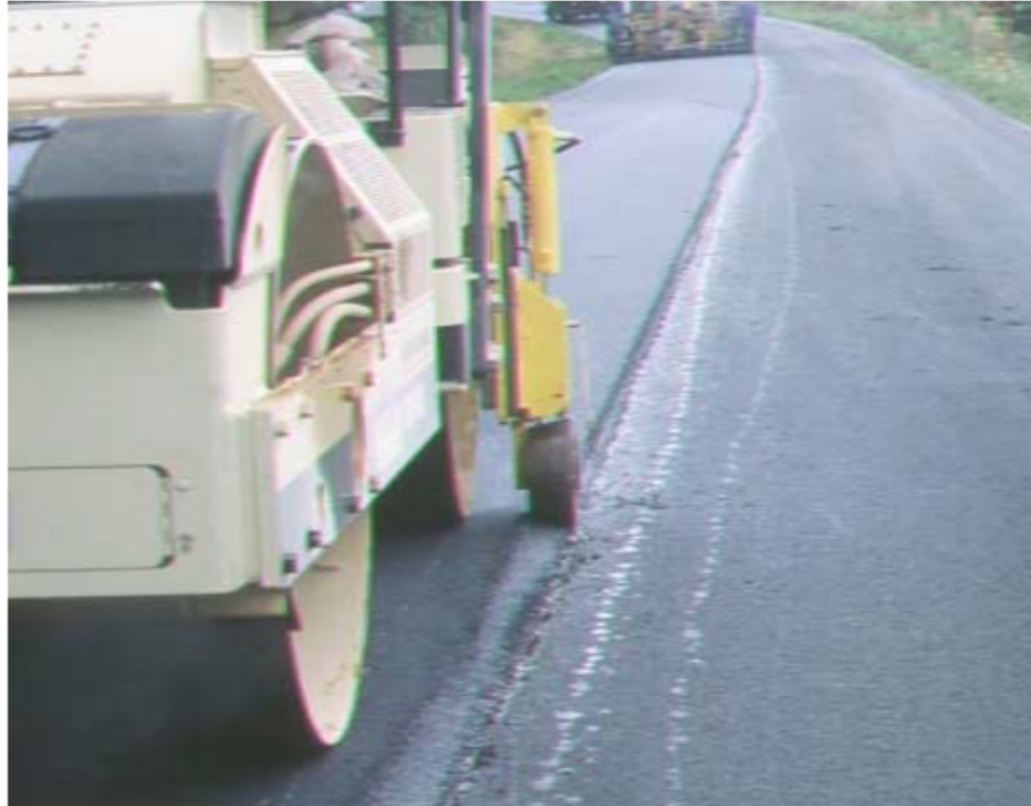
Figure 2.26: Edge restraining device mounted on a roller. (Fleckenstein 2002)
