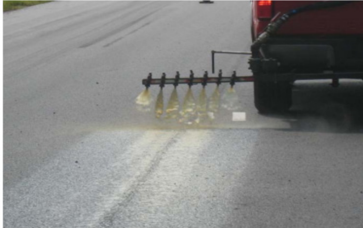
Figure 2.21: Application of Joint Bond by Pavement Technology, Inc. (Williams 2011)
