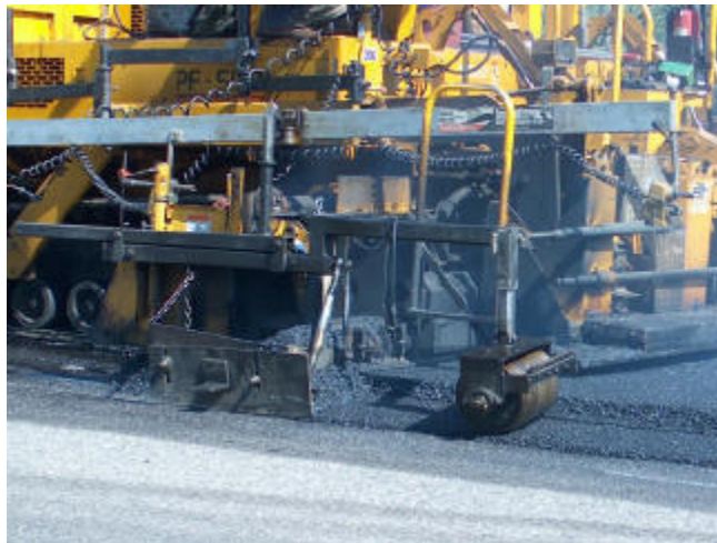
Figure 2.16: Roller attached to a paver for compaction of tapered part in notched wedge joint. ( https://www.pavementinteractive.org/ )
