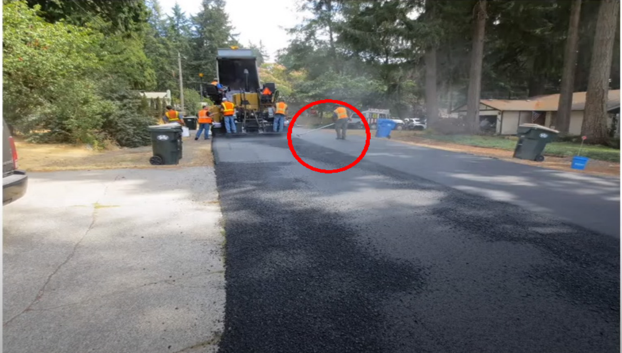
Figure 2.14: Raking of material back to the mat. ( https://www.youtube.com/watch?v=6NLURo8IBb4 )
