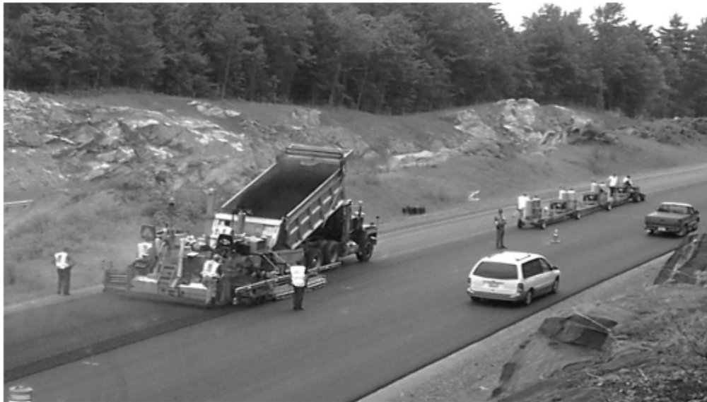
Figure 2.11: Paving with an Infrared Joint heater. (Daniel and Real, 2006)
