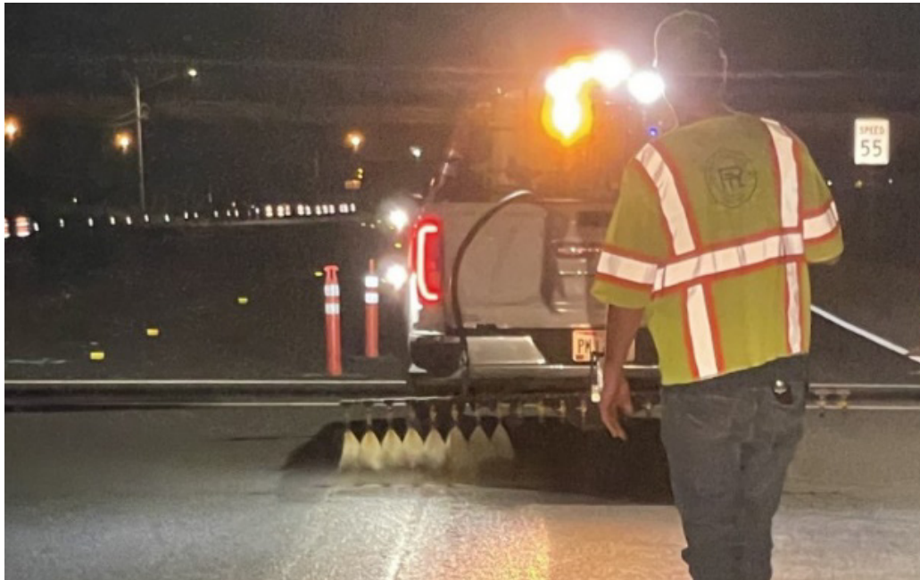
Figure 5.8: Topical emulsion applied on the OR18-McMinnville project.
