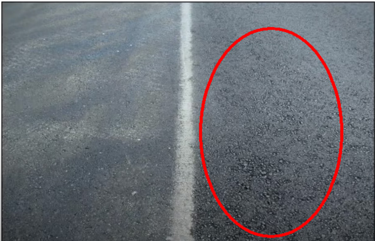
Figure 2.15: Uneven surface texture due to raking. ( https://www.youtube.com/watch?v=6NLURo8IBb4 )
