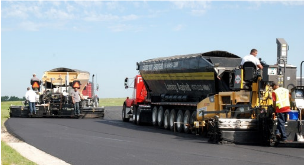
Figure 2.10 Echelon paving at GingerMan Raceway South Haven, MI. ( https://www.forconstructionpros.com )
