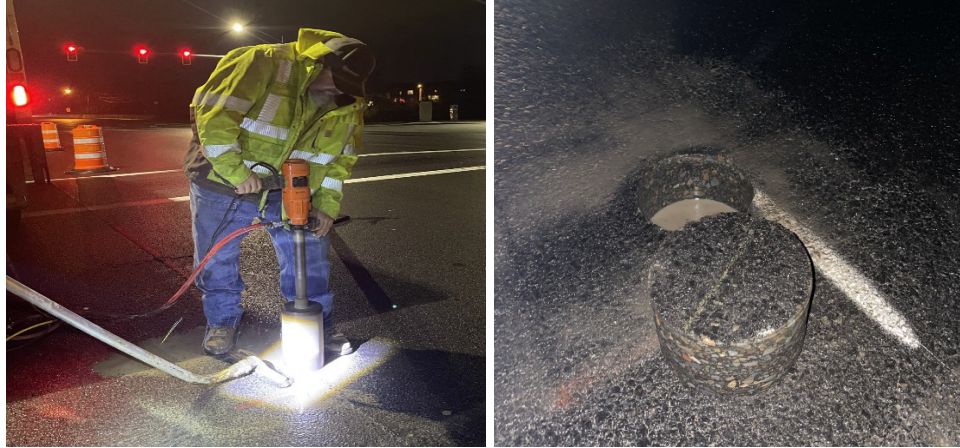
Figure 5.10: Core extracted from the pavement.
