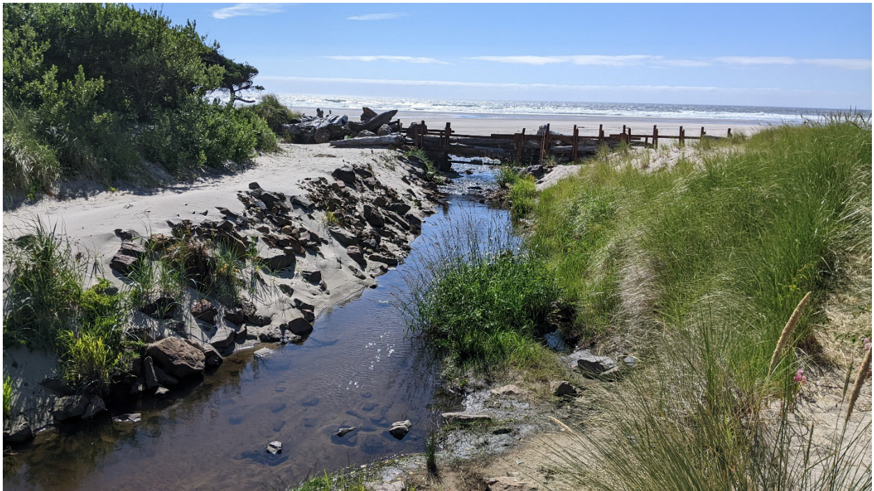
Figure 7.12: Photograph looking westward at the Saltair Creek site showing the drainage channel restoration (July 2022)
