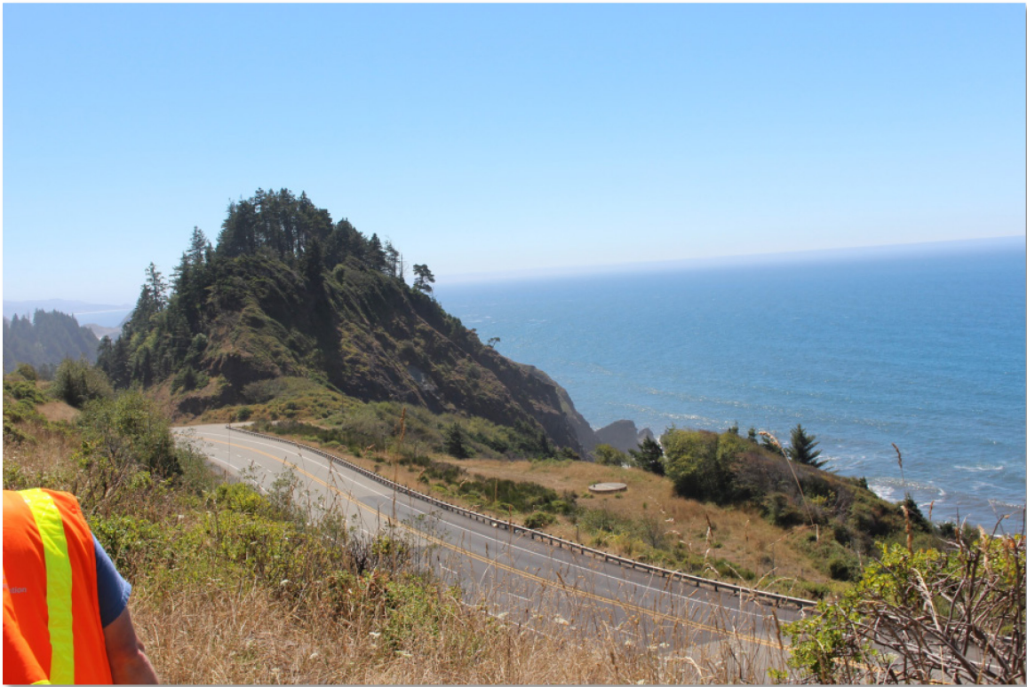
Figure 7.21: Photograph showing Hwy 101 running through Arizona Inn (facing south from the upper section of the landslide deposit). Note the freshly paved section as a repair to the creeping landslide movement (August 2016).
