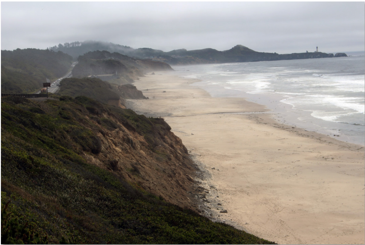
Figure 7.14: Photograph showing Spencer Creek site, facing south, with Hwy 101 shown on the left separated from ocean by the crumbling coastal seacliff (Near MP 134, Aug 2016).
