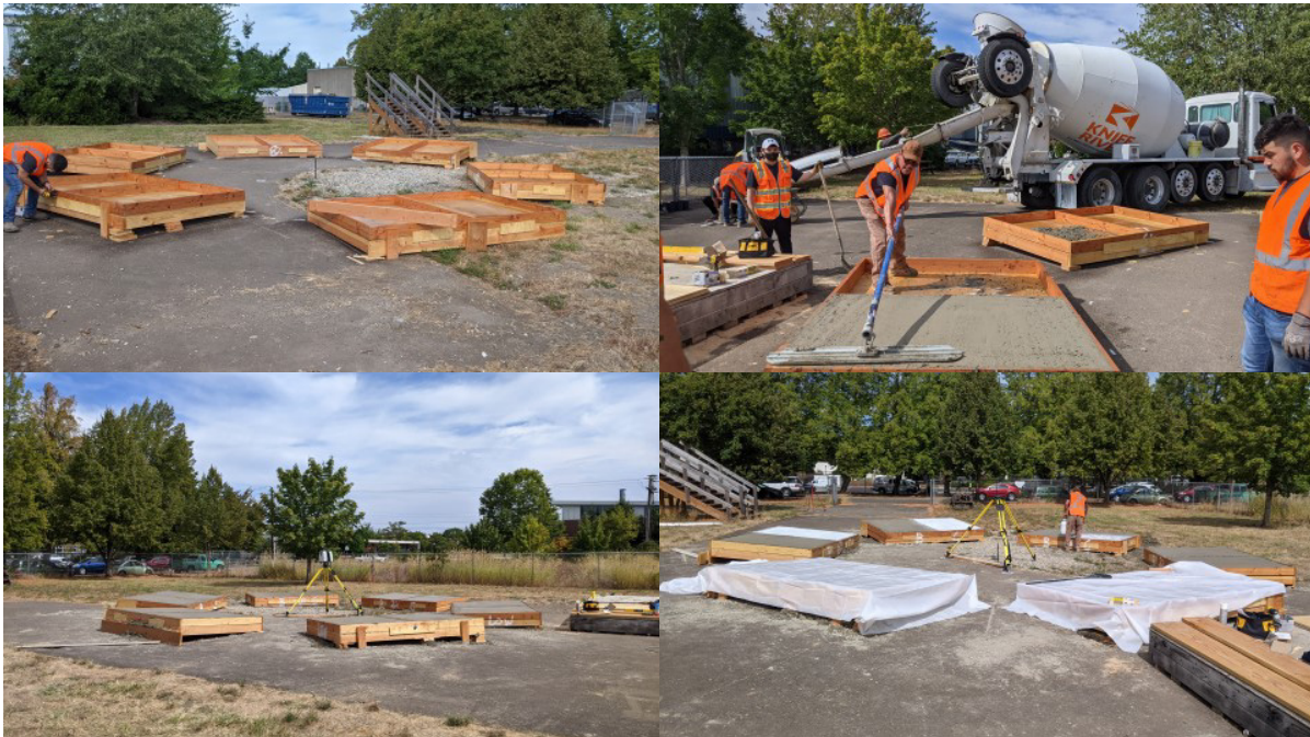
Figure 6.2: Ramp construction and survey configuration of the lab test for the concrete evaluation.
