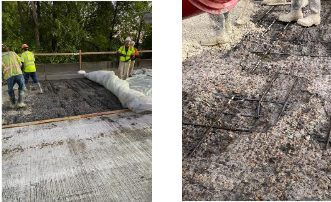
Figure 2-4 Hydro demolition of an Oregon DOT bridge deck prior to HESC placement
