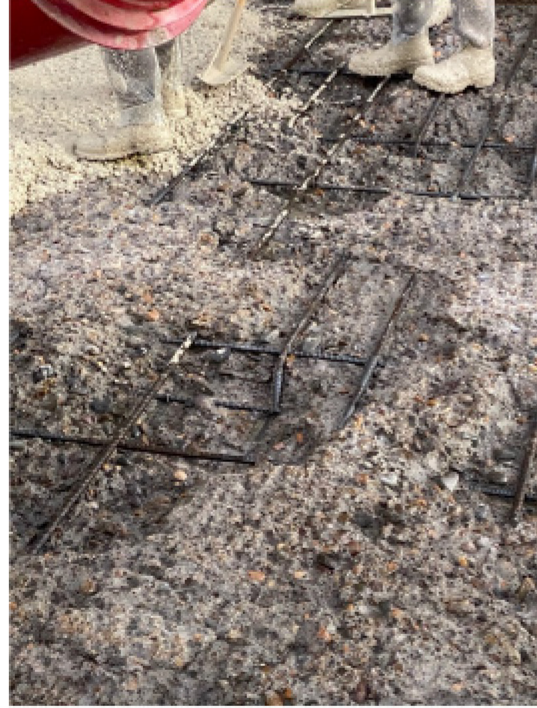
Figure 4-31 Hydrodemolition preparation of Yamhill Crossing bridge deck (BR# 08492), July 26, 2020.
