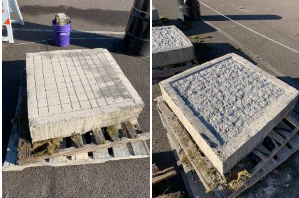
Figure 3-5. Slab saw cut at a six-inch spacing (left) and removed with demolition hammer (right)
