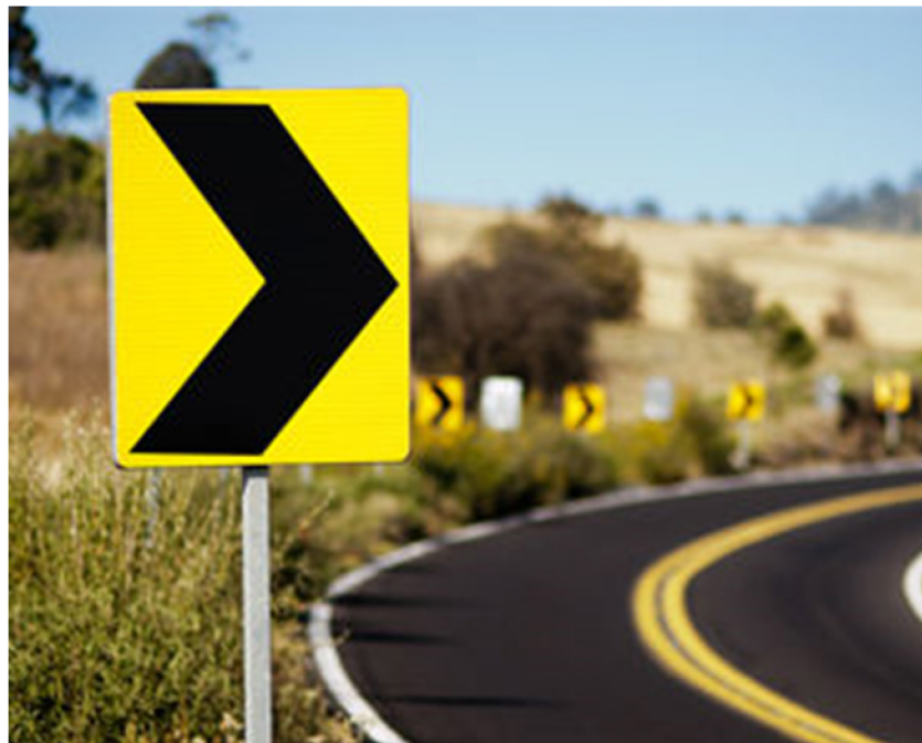
Figure 2.7 Chevron signage (WSDOT, 2019)
