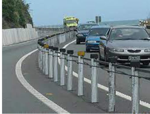
Figure 2.1: Cable Median Barrier along the midsection of the roadway
