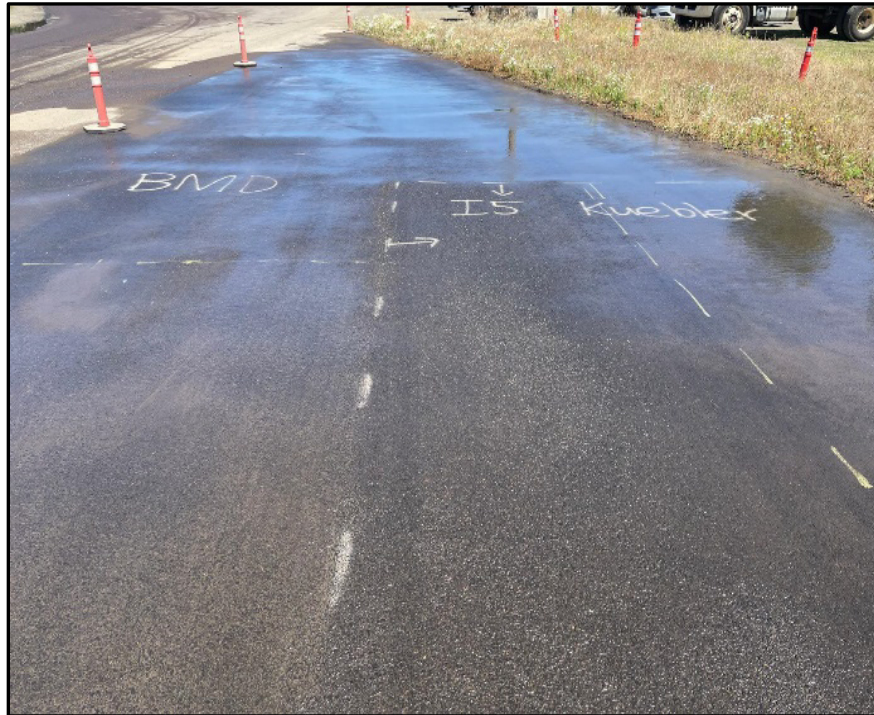
(e) Final test sections with markings
