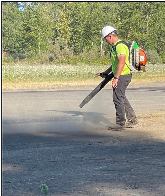
(a) Dust removal from the adjoining pavement
