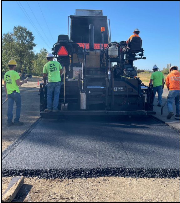
(c) Paving process
