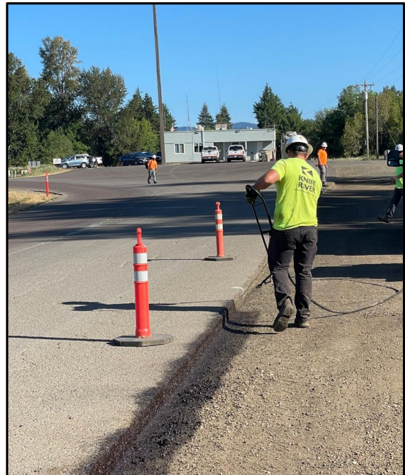
(b) Application of tack coat on the old pavement
