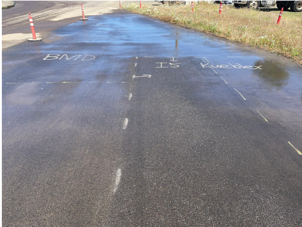
Figure 6.3: Cleaned test section (BMD and volumetric mixes)
