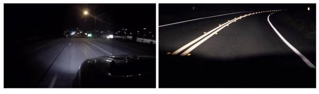
FIGURE 2.7: CONTRAST BETWEEN LOW RETROREFLECTIVITY PAVEMENT MARKINGS TO THE LEFT AND HIGH RETROREFLECTIVITY MARKINGS TO THE RIGHT (GOOGLE, 2021)
