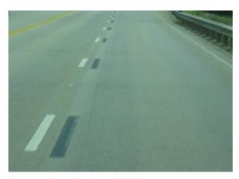
FIGURE 2.5: MASKING BEING USED TO COVER UP PAVEMENT MARKING (NCHRP, 2013)
