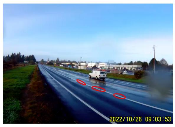
FIGURE 5.4: PAVEMENT MARKING REMOVAL ON US 101, WARRENTON, OR
