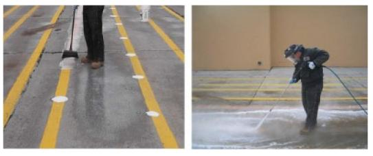
FIGURE 2.4: APPLICATION OF CHEMICAL REMOVER TO THE LEFT AND REMOVAL TO THE RIGHT (CHO ET AL., 2013)
