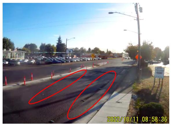
FIGURE 5.1: PAVEMENT MARKING REMOVAL ON US 20, ALBANY, OR
