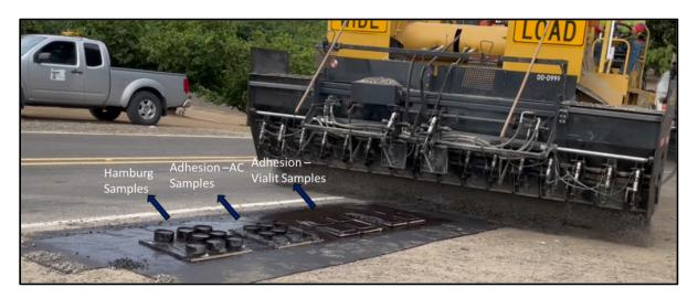
Figure 3.19: Woodburn chip seal sampling section
