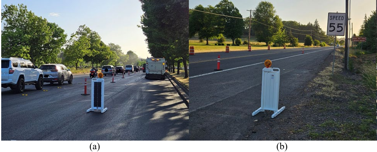
Figure 6.2: Location Beacon Deployments Onsite: Start-of-Workzone (a), and End-of-Workzone (b)
