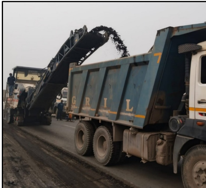
Figure 2.2. Milling of asphalt pavement
